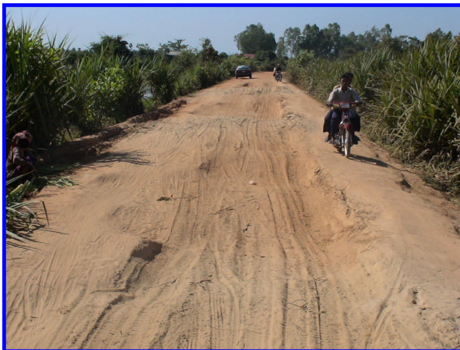
Figure 1 – A donor funded project gravel road within 2 years of maintenance cessation (dry season and impassable by motor car!)
