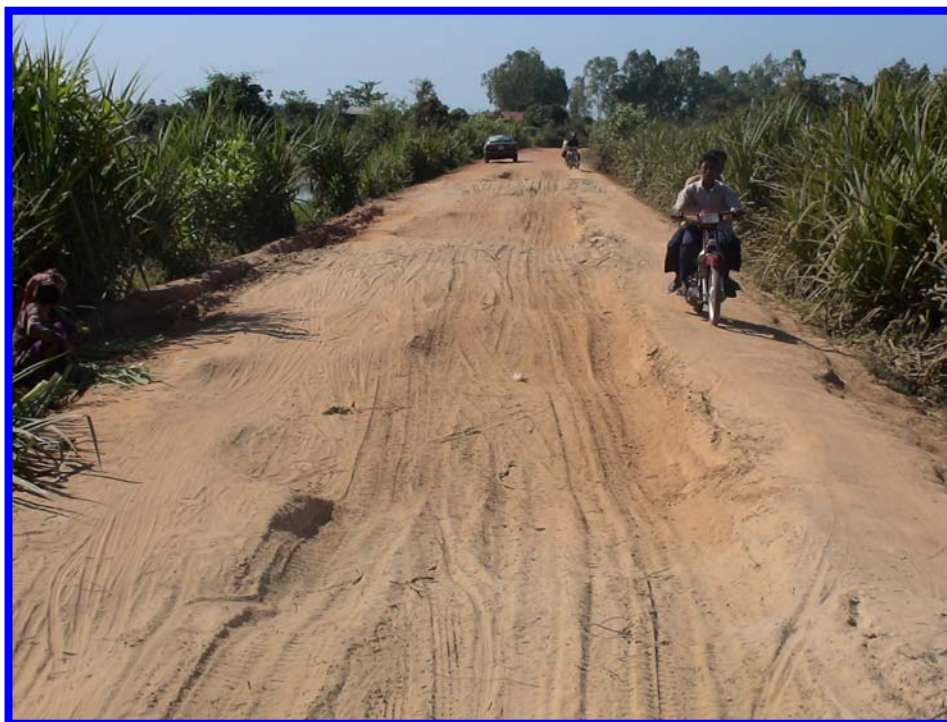
Figure 3 - A donor funded project gravel road within 2 years of maintenance cessation (dry season and impassable by motor car!)
