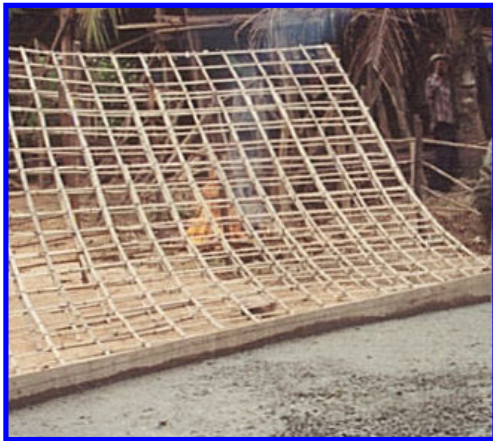
Photos 2 and 3 – Bamboo Reinforced Concrete road
