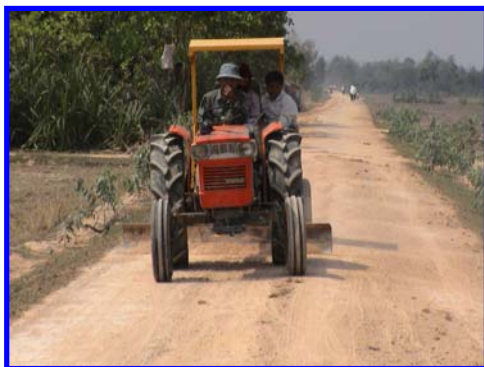
Photos 8 and 9 – DTW designed towed grader for road maintenance
