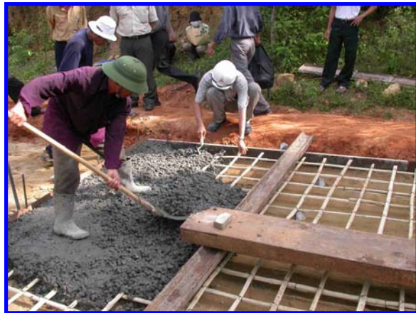
Photos 2 and 3 – Bamboo Reinforced Concrete road
