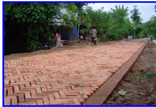
Photos 6 and 7 – Rice husk burnt clay brick production and paving
