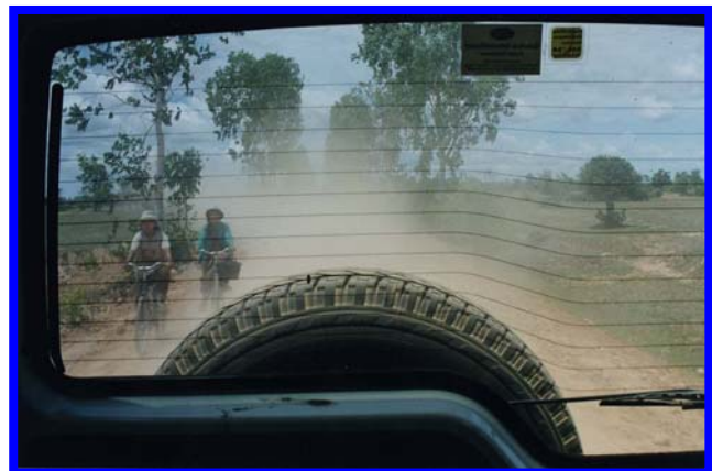
Figure 2.1 Dust emissions from gravel road in the dry season
