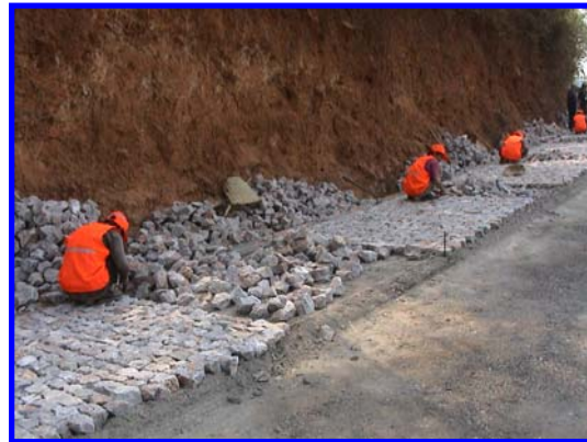
Photos 4 and 5 – Hand quarried stone and Cobble Stone Paving
