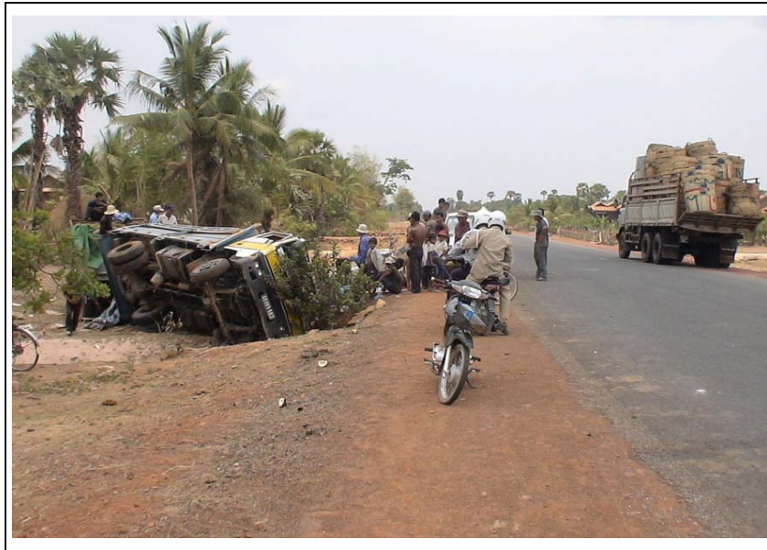
Figure 11 - Deep irregularities in shoulders can cause vehicles to roll over if they veer off the carriageway.
