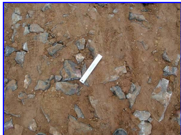
Photograph A2-3 and A2-4: Road-base under construction: urban road in BMC province (Clayey soil was used to fill voids between hand packed stone)
