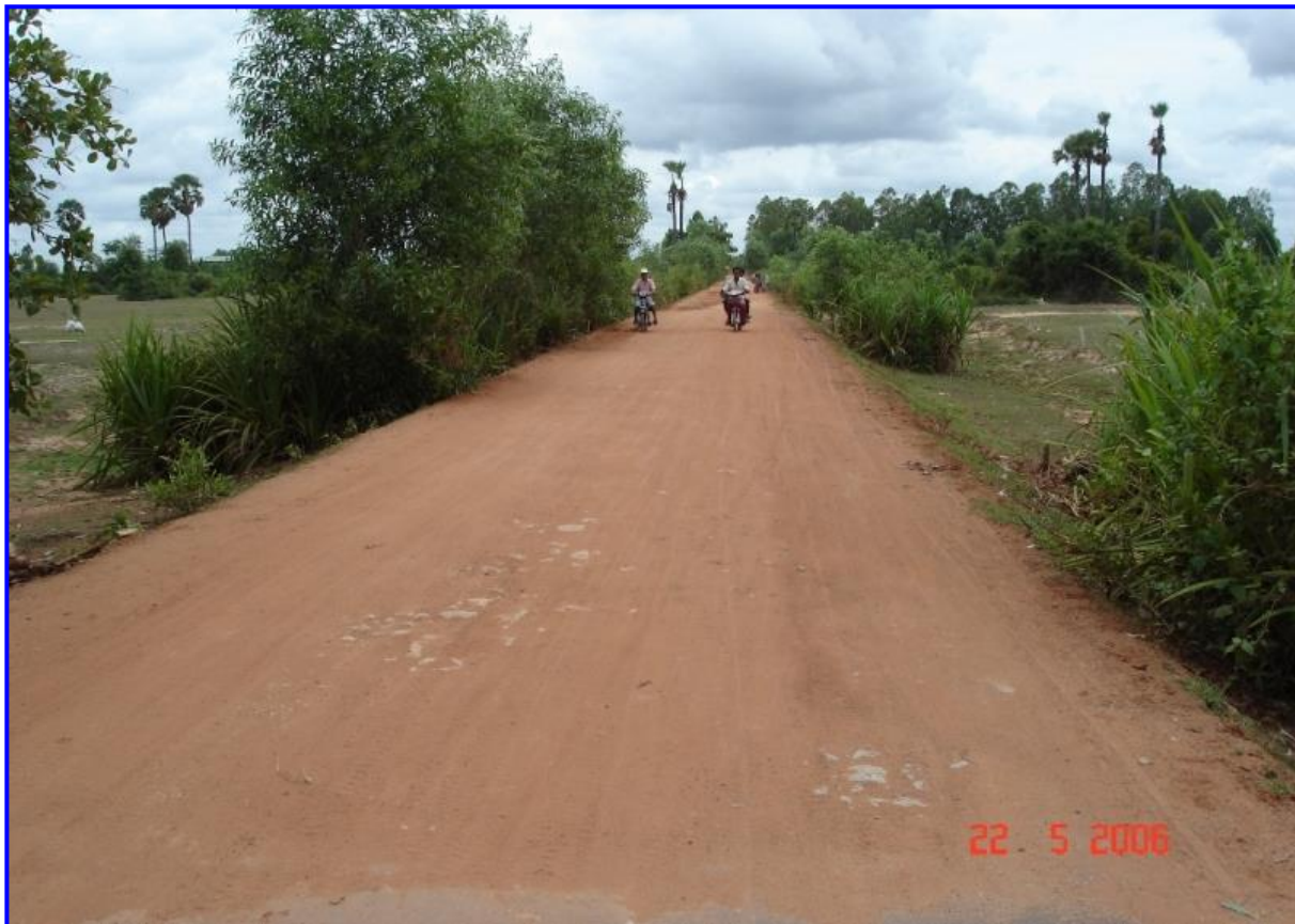
Figure 7.3: Trial Section 10: Gravel surface over hand packed stone
