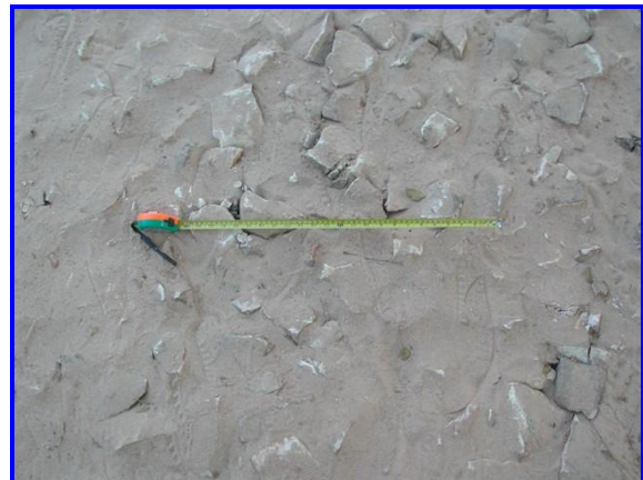
Photograph A2-1 and A2-2 – Road in front of the Provincial Department of Rural Development Siem Reap Town (Fine sandy-clay was used to fill voids in between stone aggregate)
