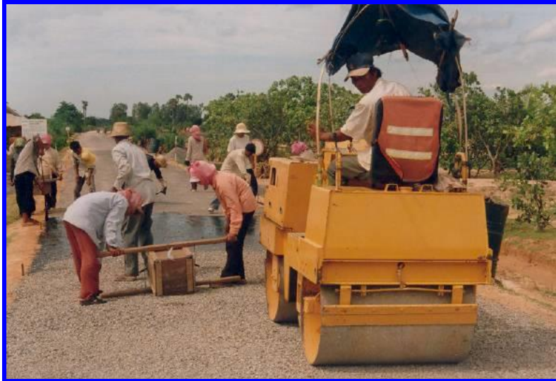
Figure 1.2: Puok Trials Construction Works
