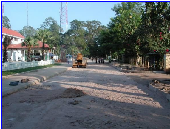
Photograph A2-1 and A2-2 – Road in front of the Provincial Department of Rural Development Siem Reap Town (Fine sandy-clay was used to fill voids in between stone aggregate)
