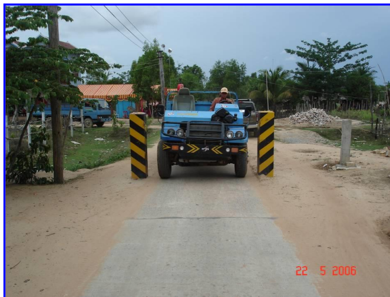
Figure 4.1: Vehicle side-restriction barrier, Puok Market Trials
