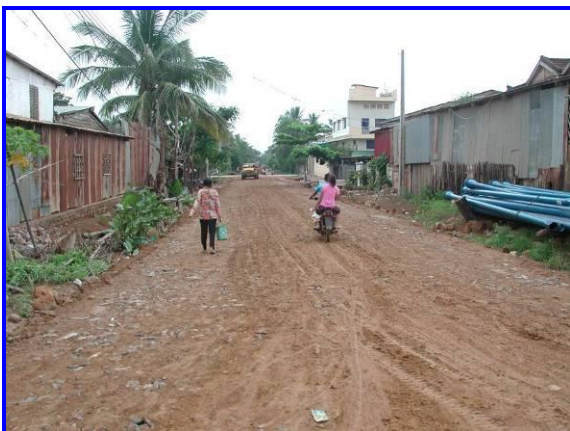
Photograph A2-3 and A2-4: Road-base under construction: urban road in BMC province (Clayey soil was used to fill voids between hand packed stone)
