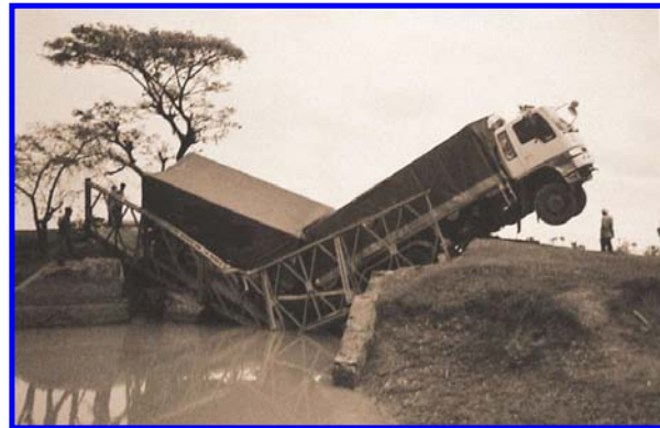
Image 2 – Overloaded truck damages bridge on a secondary road.
