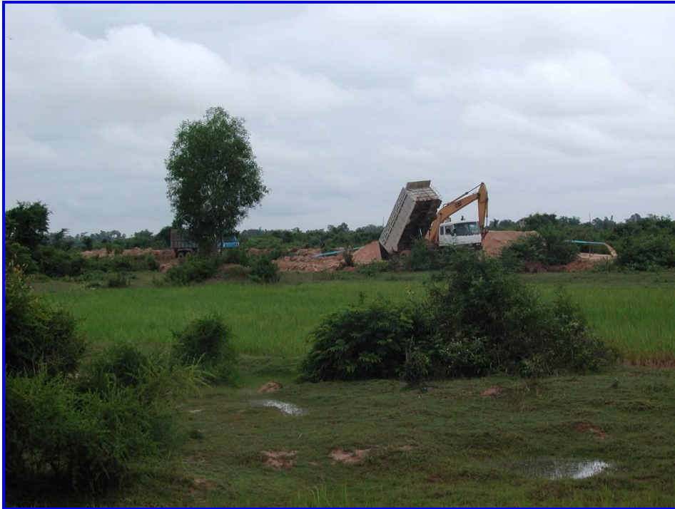
Sand extraction quarry
