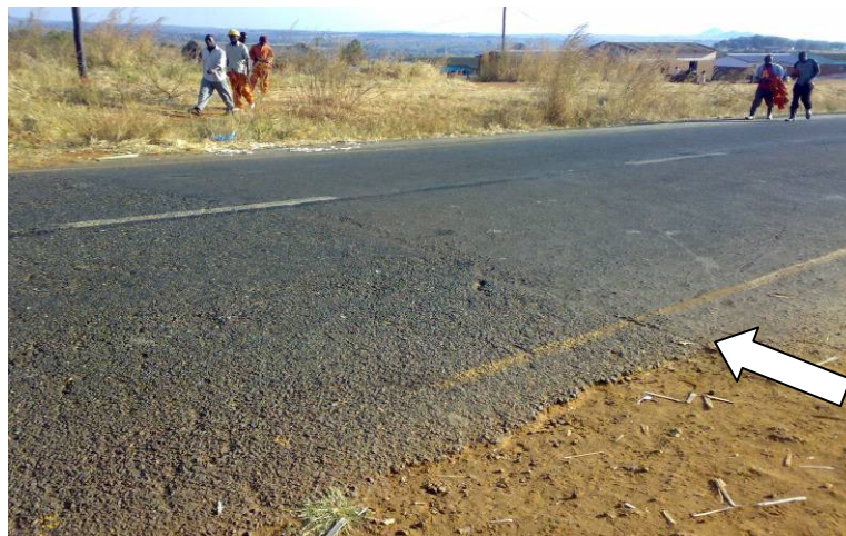
Figure 5: Ntchisi Conventional (4 yrs old) and Low Volume Sealed Road (9 yrs old) Road Sections connection
