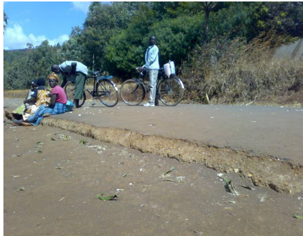
Figure 2: Typical LVSR (6 yrs old) – 150mm Gravel placed direct on existing earth road
