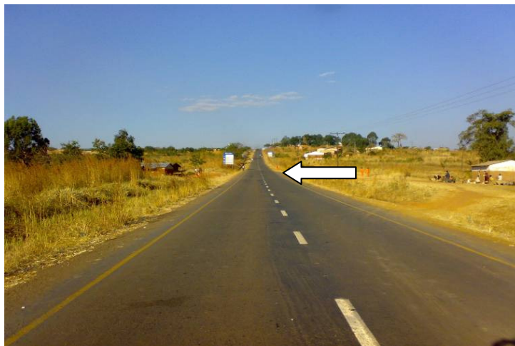
Figure 4: Conventionally Upgraded (4 yrs old) and Low Volume Sealed Road (9 yrs old) Road Sections connection
