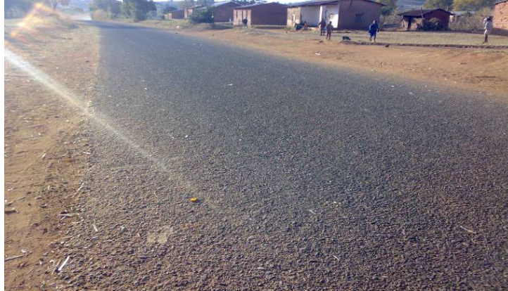
Figure 3: Low Volume Sealed Road after 9 years being in use
