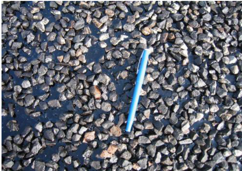
Bitumen filled seal
