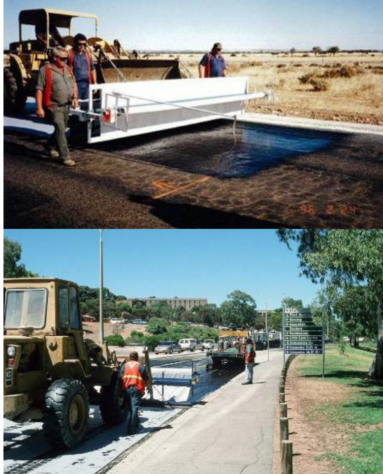
Installation of fabrics
