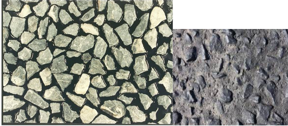
Typical spread of aggregate for a Cape Seal
