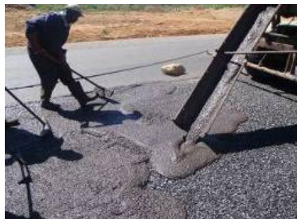
Hand-spreading of slurry
