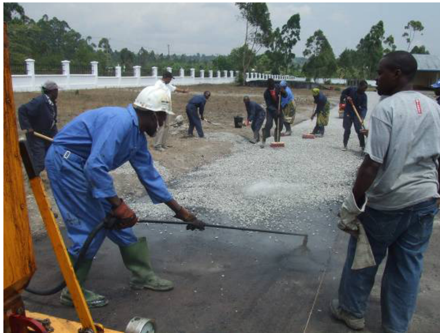
Continuous operation of spraying binder and spreading chippings
