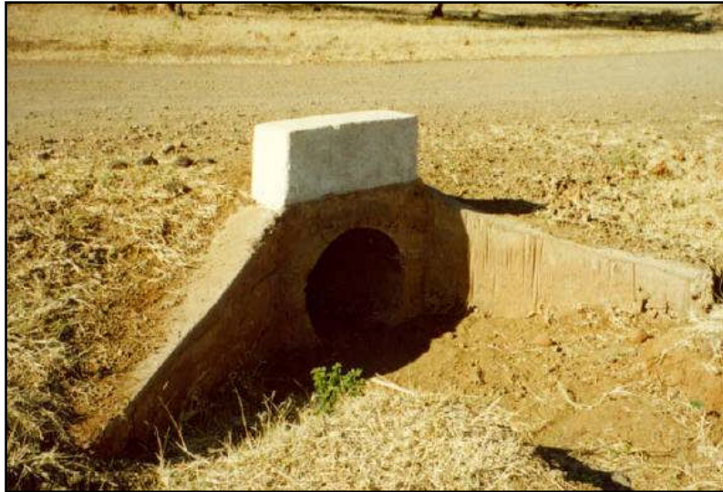
Figure 3.5 Culvert head stone outside main running lanes
