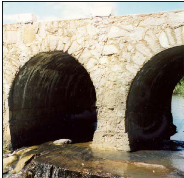
Figure 4.11 Large bore arch culverts
