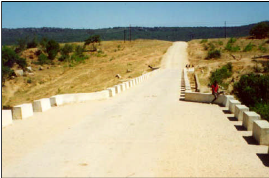
Figure 3.4 Guide stones narrowing road width
