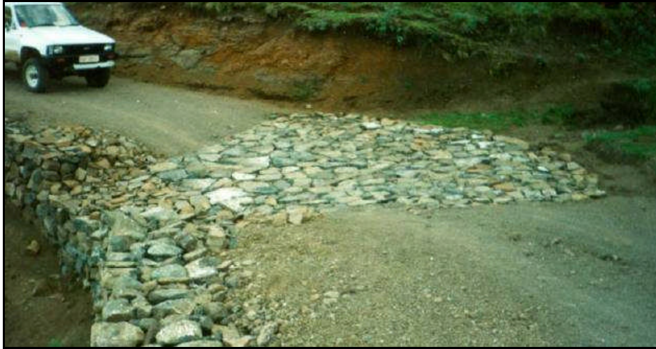
Figure 4.3 A basic hand packed stone drift
