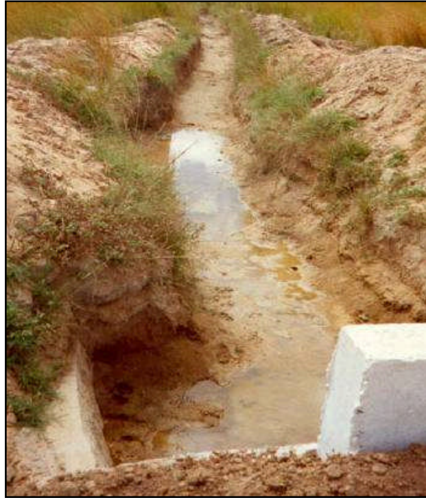
Figure 5.8 Long culvert outfall
