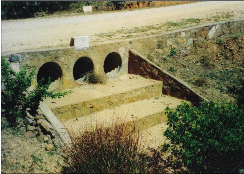
Figure 4.5 A three barrel corrugated steel culvert with stepped outfall apron
