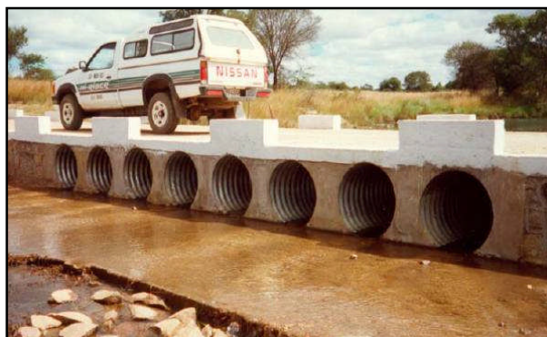
Figure 4.8 Downstream protection to a vented ford
