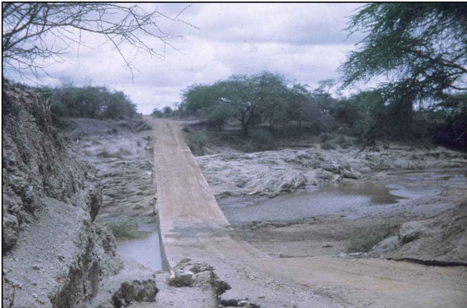
Figure 4.9 Concrete vented causeway
