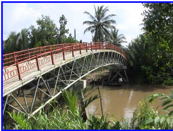
Figure 1.1 Steel lattice bridge for motorcycle traffic
