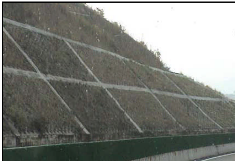
Figure 7.16 Hybrid retaining wall
