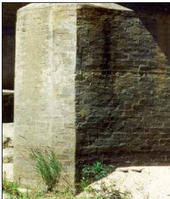
Figure 7.32 Bricks in a bridge pier
