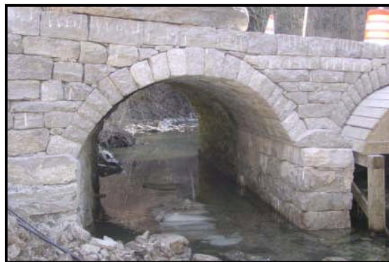
Figures 7.18 Dry stone masonry culvert extension works – Dry stone Conservancy, USA
