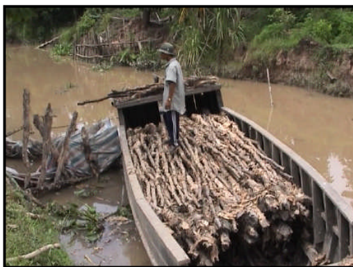
Figure 7.38 Timber poles for piles (not covered by this guideline) for a concrete box culvert in very soft ground
