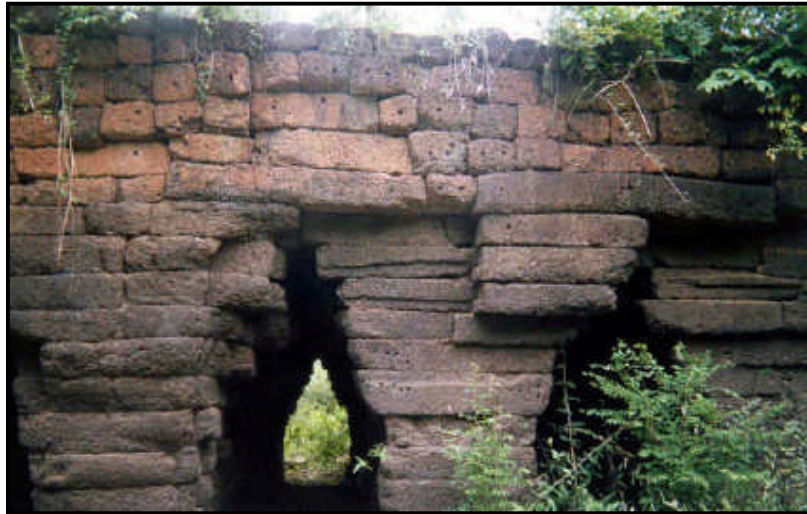
Figure 7.1 Dry jointed, multiple opening, cantilevered laterite stone culvert approximately 1,000 years old and still in service.
