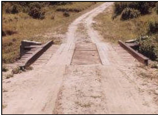
Figure 7.42 Timber decked bridge
