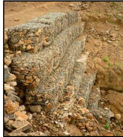
Figure 7.19 Gabions supporting a road on a steep slope
