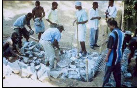
Figure 7.21 Filling gabion baskets
