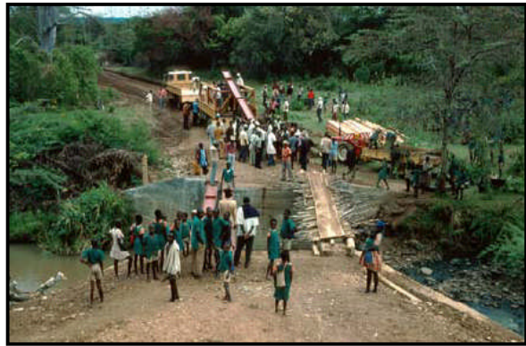
Figure 7.33 Steel beams being moved into position using labour methods without the use of cranes ready for completion with a timber deck
