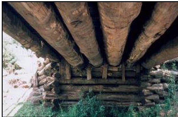
Figure 7.43 Log abutments & deck
