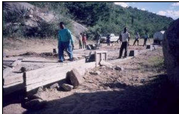
Figure 7.51 Concrete drift in construction
