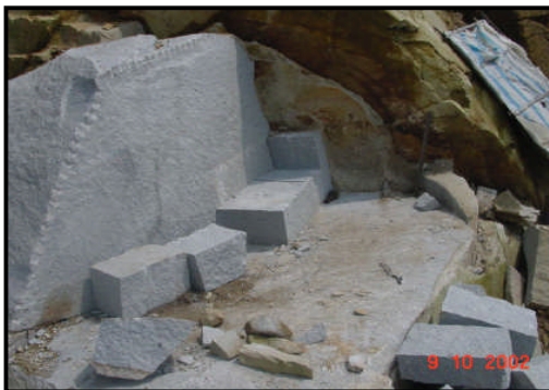
Figure 7.5 Hand quarried granite stone blocks
