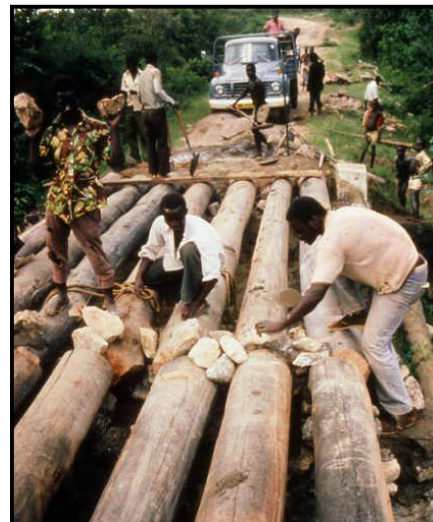
Figure 7.39 Timber poles as deck beams of a twin span bridge
