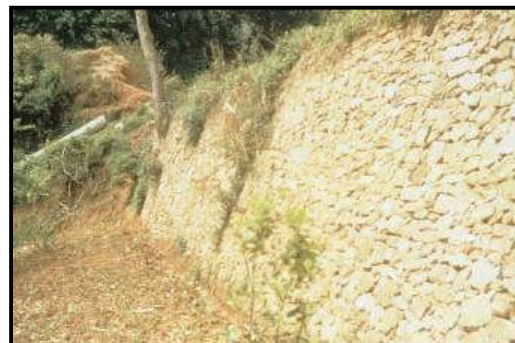
Figure 7.12 Dry stone wall supporting road embankment
