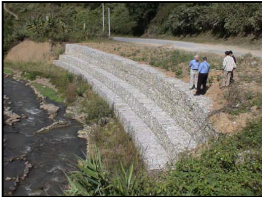
Figure 7.22 Gabion retaining wall used as river bank protection
