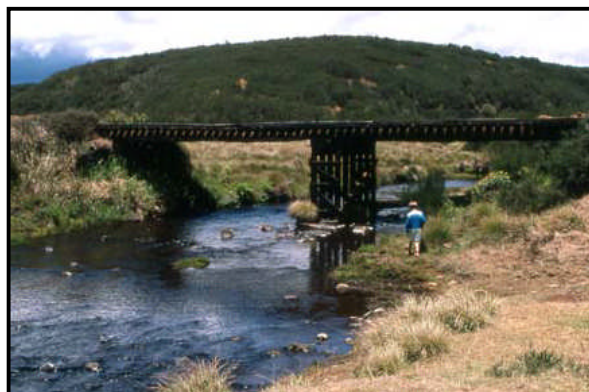
Figure 7.36 Timber bridge deck, pier and abutments
