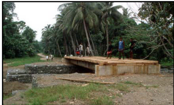
Figure 7.34 Timber deck on recycled steel beams
