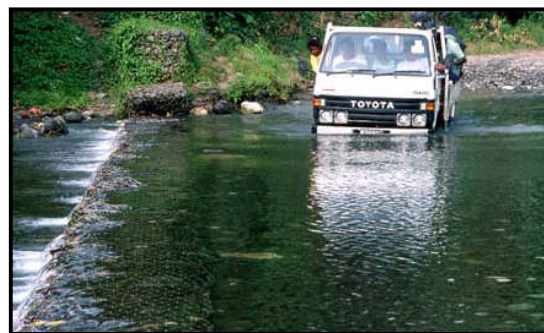
Figure 7.25 Gabion river crossing
