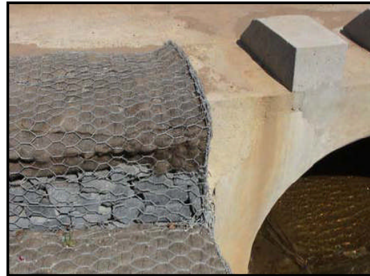
Figure 7.23 Natural fibre matting inserted in gabion protection works to encourage rapid growth of vegetation cover
