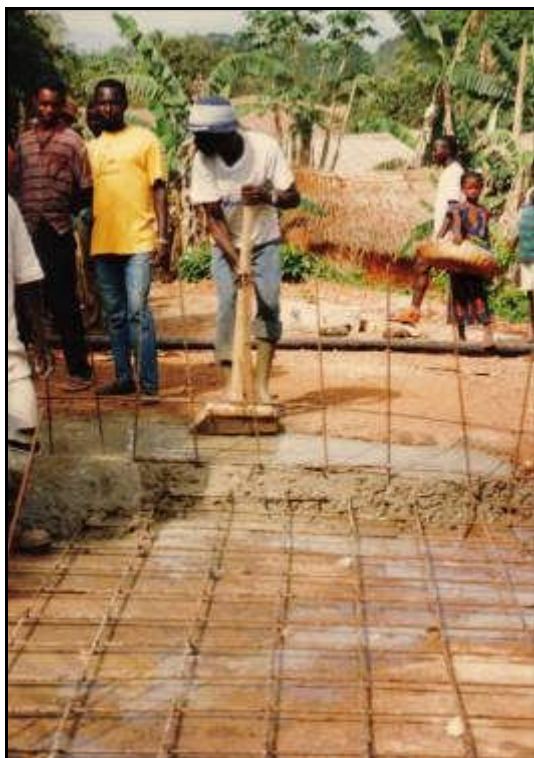
Figure 7.52 Reinforced concrete slab
