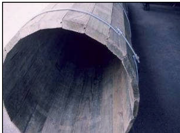
Figure 9.13 Timber stave culvert
