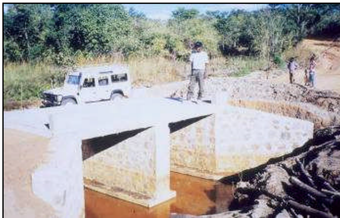
Figure 8.53 Reinforced concrete deck on masonry abutments and pier
