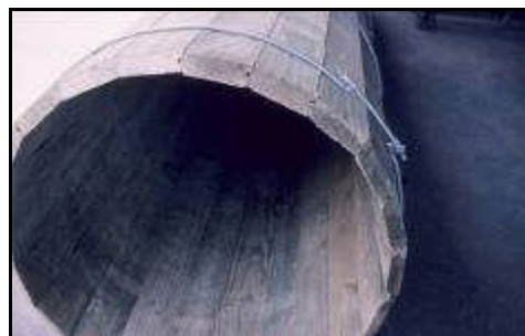
Figure 8.17 Timber barrel culvert
