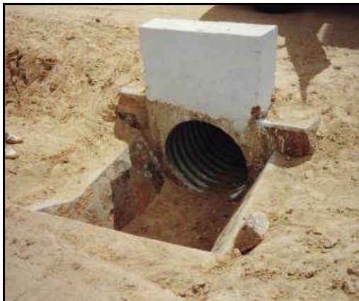
Figure 8.26 Drop inlet on stream culvert
