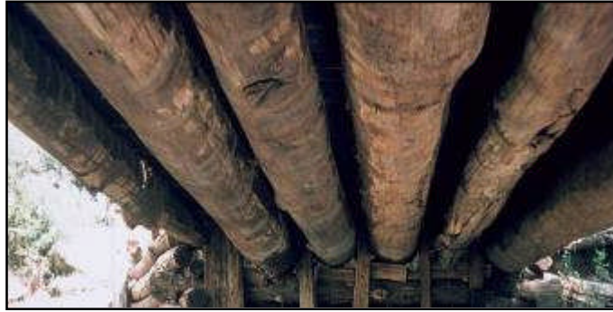
Figure 8.58 Log stringers from underside of bridge deck
