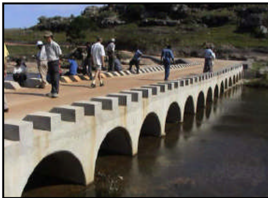
Figure 8.62 Raised kerbs on a vented causeway allow water to pass over the structure with minimum disturbance, but provide protection from vehicles driving off the structure.
