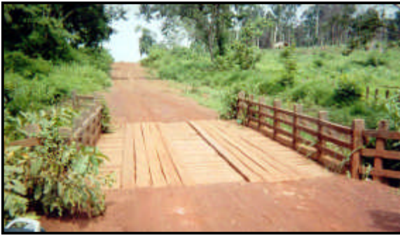
Figure 8.63 Timber bridge with handrails
