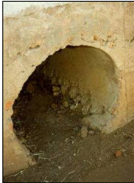
Figure 8.21 Cast in situ culvert
