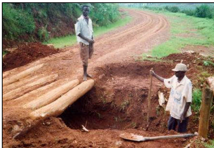
Figure 8.19 Timber pole culvert during reconstruction
