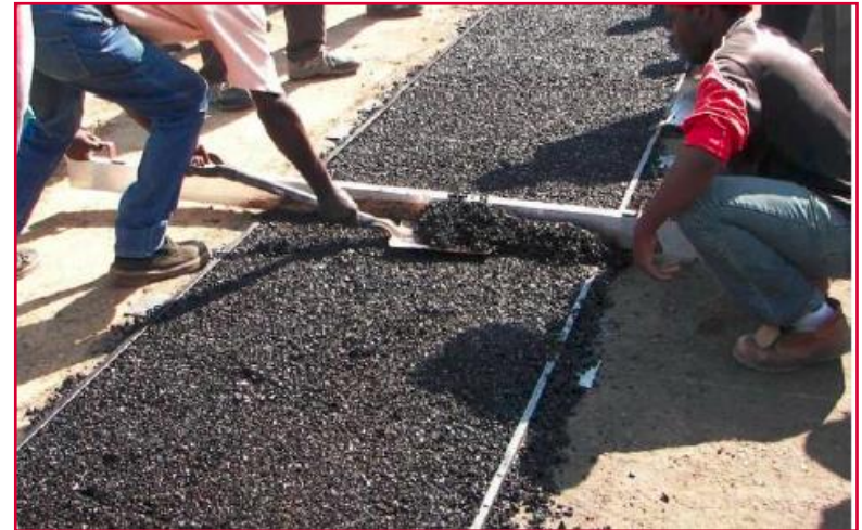
Thin cold mix asphalt
