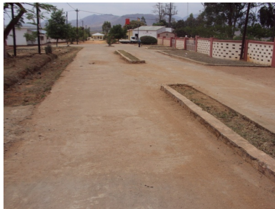
Cement-grouted stone+cement mortar screed
