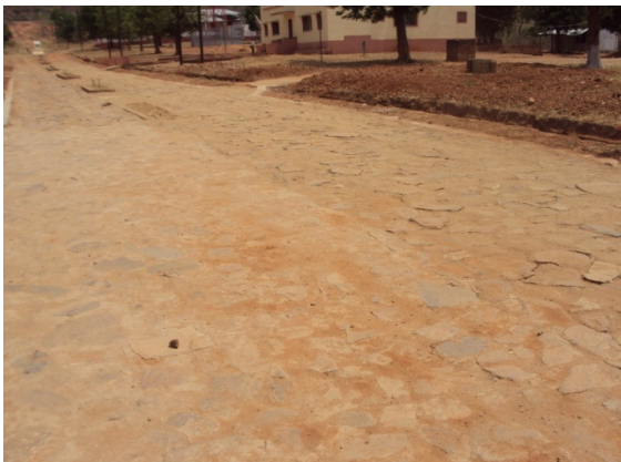
n° 11: Cement-grouted stone on LHS
