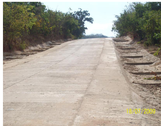
Photo n° 14: After intervention, July 2009
