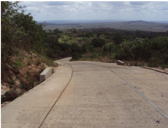
Photos n° 15: Section as at October 2010 - no tensile cracking observed
