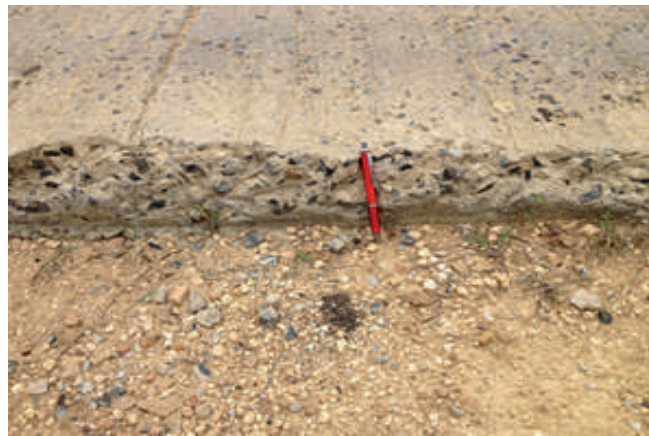
Figure 15-9: Concrete strip road with dangerous edge drop
