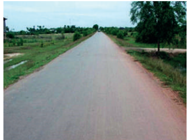
Figure 16-7: Paved road option (Higher construction costs, lower maintenance and road user costs)
