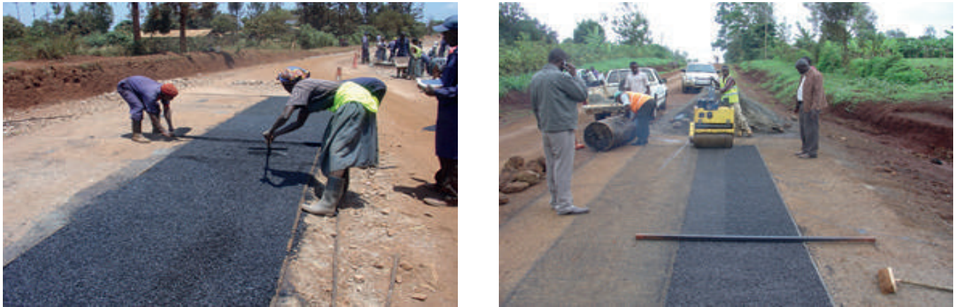
Figure 15-6: Levelling and compaction of Cold Mix Asphalt
