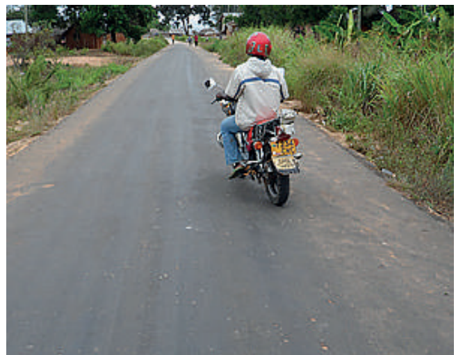
Figure 2-8: Low volume paved road
