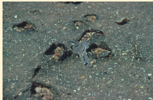
Figure 6-9: Mechanism of soluble salt damage to bituminous surfacings
