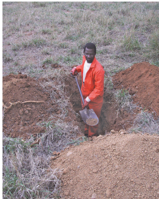
Figure 5-3: Test pits for LVRs are commonly excavated using labour
