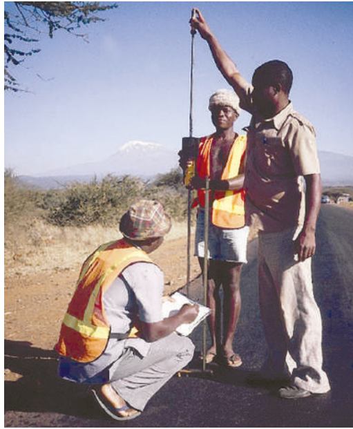
Figure 5-1: Carrying out a DCP test on a paved road
