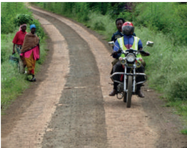
Figure 2-7: Concrete strip road
