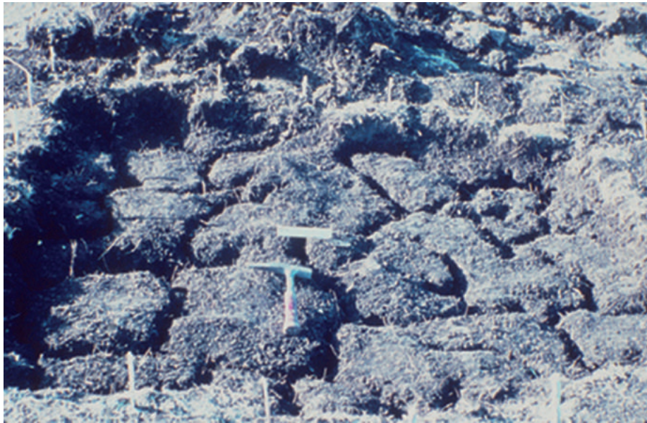
Figure 6-2: Cracking on expansive clay
