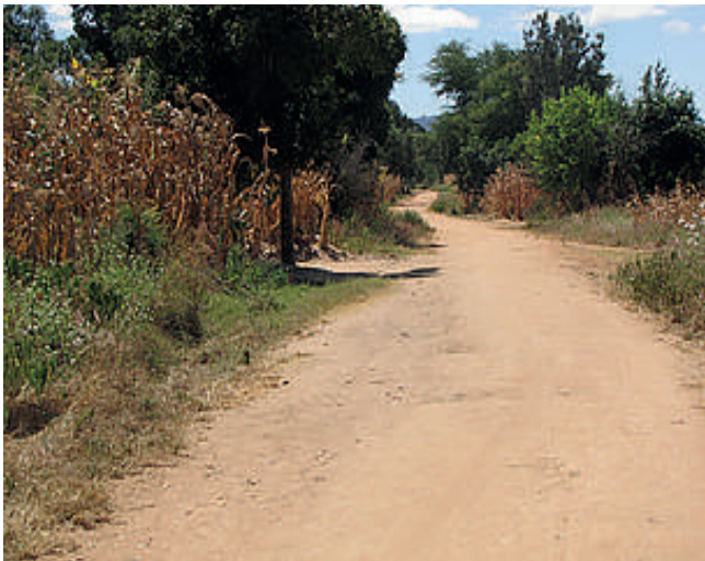
Figure 2-5: Non-engineered natural soil track/road
