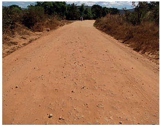
Figure 2-6: Engineered gravel road
