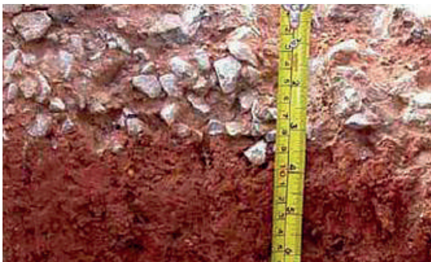
Figure 7-10: Crushed stone armouring on laterite
