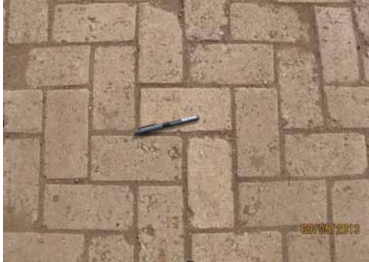
Photo 7-3: Example of concrete brick paving (Herringbone pattern)
