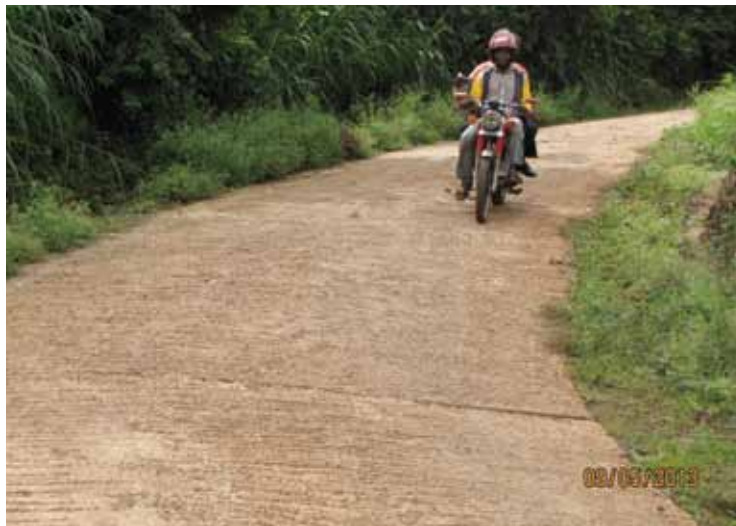
Photo 7-5: Example of reinforced concrete surfacing
