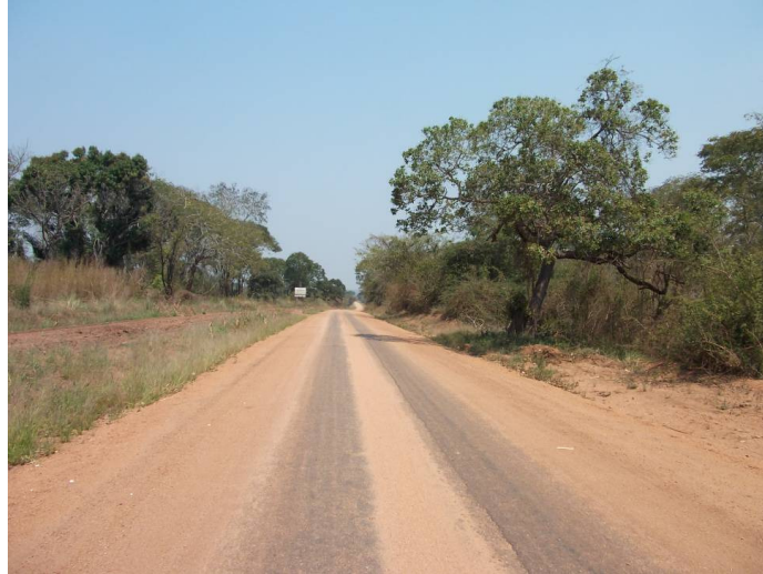
Figure 2: Otta seal section with 1.2L/m 2 binder
