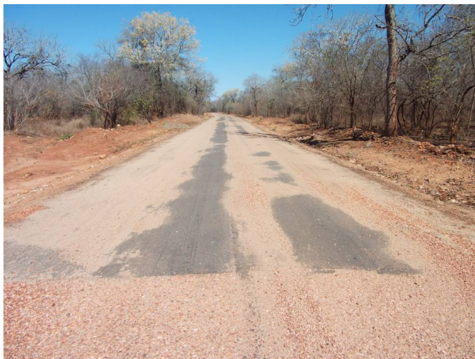
Figure 3: End of Otta seal and beginning of sand seal
