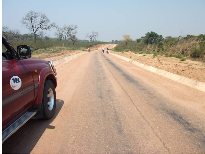
Figure Error! No text of specified style in document.1: Otta seal surfacing in curing process
