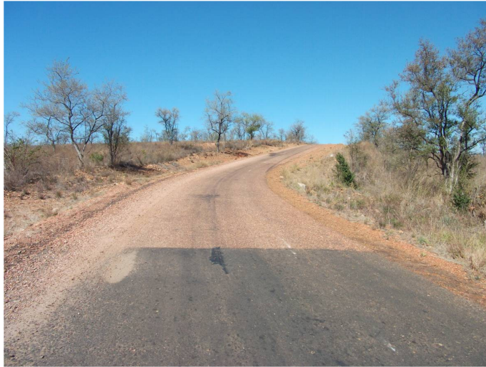
Figure 1: Single Otta seal with sand seal, Double Otta seal and 1 ½ Otta seal
