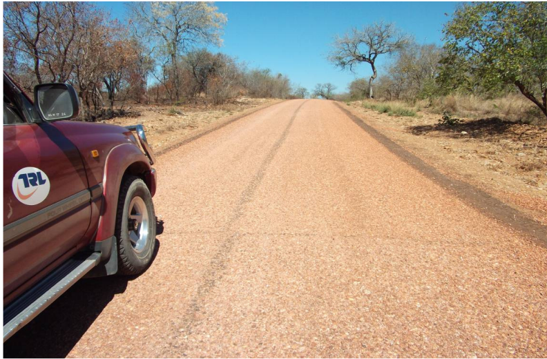
Figure 2: End of section with 1.6L/m 2 binder and beginning of section with 1.4L/m 2
