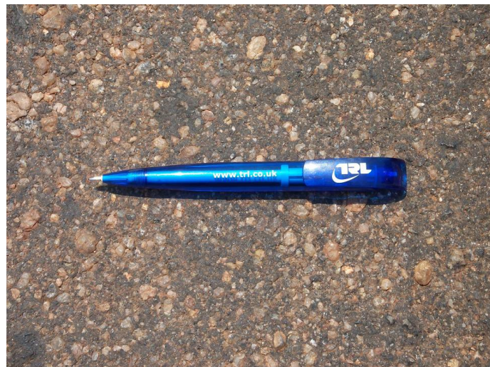
Figure 3: Otta seal surfacing with 1.2L/m 2 binder
