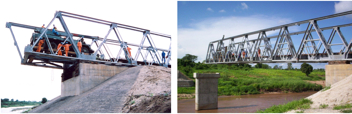
Photos 4 and 5 – Cantilever Construction
