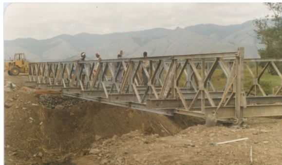
Photo 2 – Typical Panel Bridge
