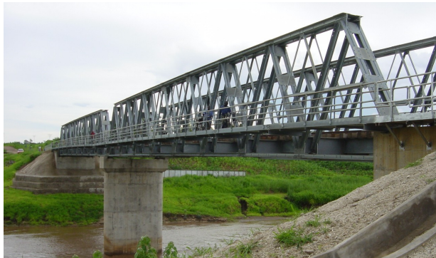
Photo 1 – Typical Truss Bridge
