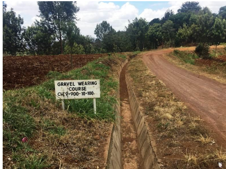
Figure 5: Grave wearing course section, with section identification marker
