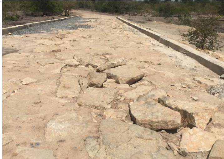
Figure 3: Hand-packed stone section
