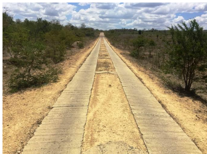
Figure 2: Concrete strip section
