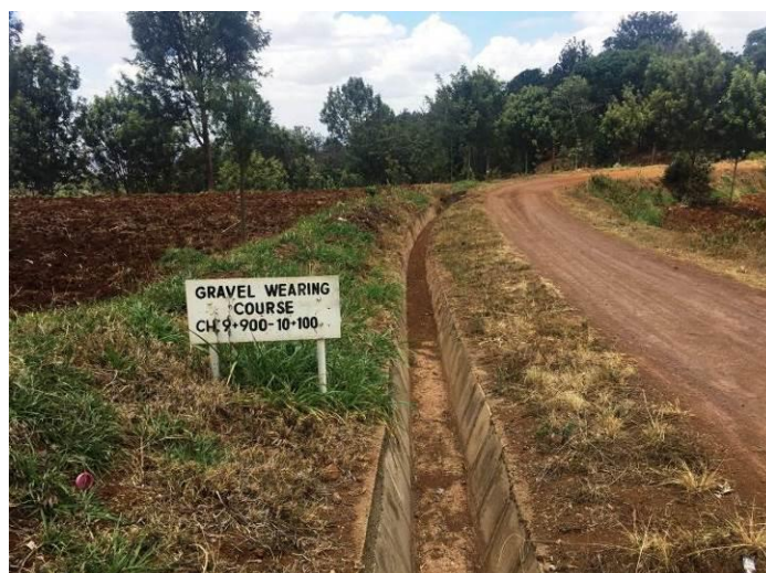
Photo A6: Gravel Wearing Course section
