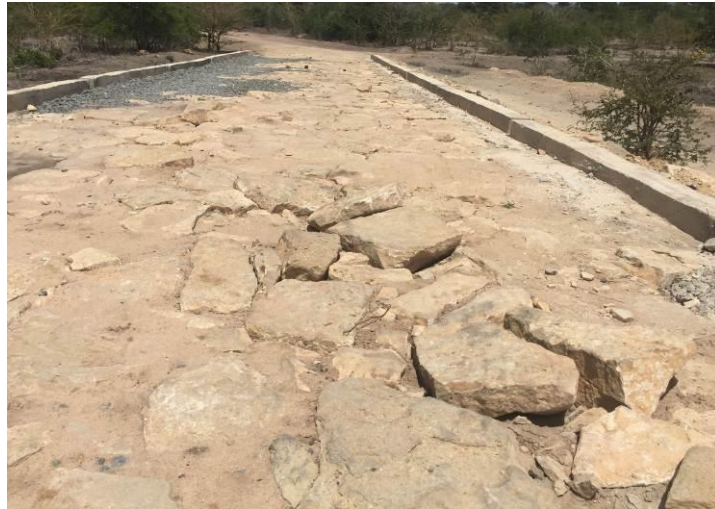
Photo 3: Hand-packed stone section
