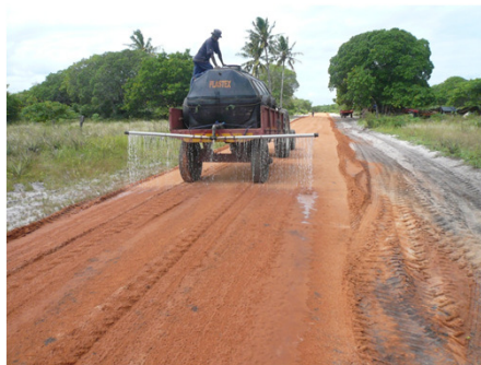
Construction of subgrade (half widths) using imported red sand
