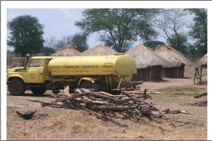
Contractor's site camp
