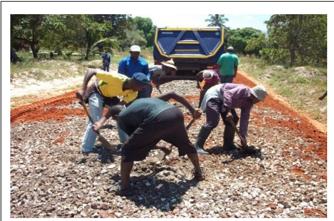
Construction of armoured base
