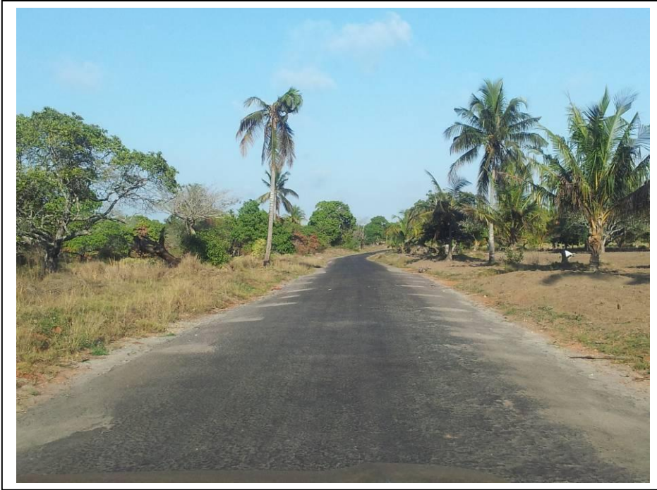
Sand seal on armoured sand base
