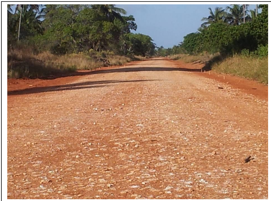
Armoured sand base
