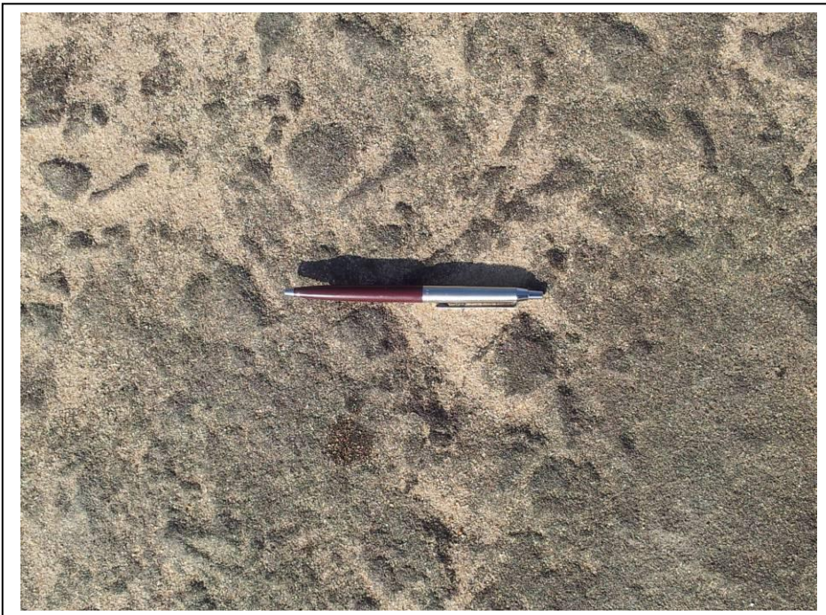
Amalgamated surfacing (sand seal)
