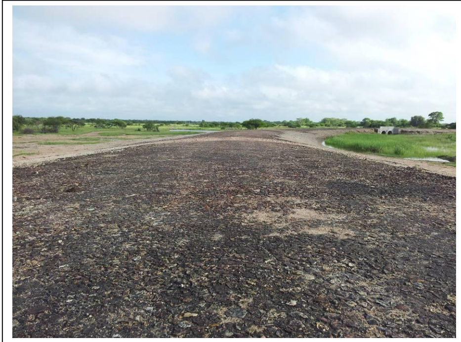
Armoured and blended sand/clay base
