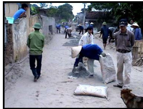
Plate 4 "Spotting" and then breaking bags prior to spreading
