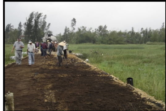
Plate 3 Final hand raking of bitumen emulsion-sand mix
