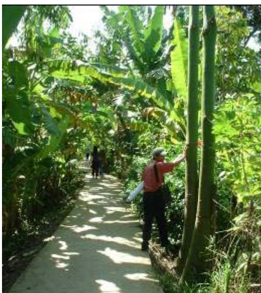
A concrete slab village road in Vinh Long province
