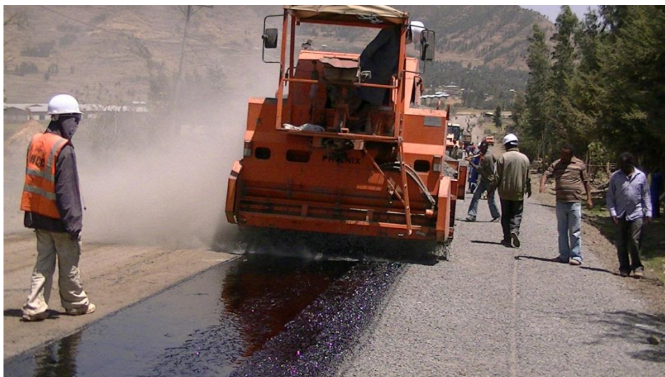
Figure 4-3 Self-propelled chipspreader in operation
