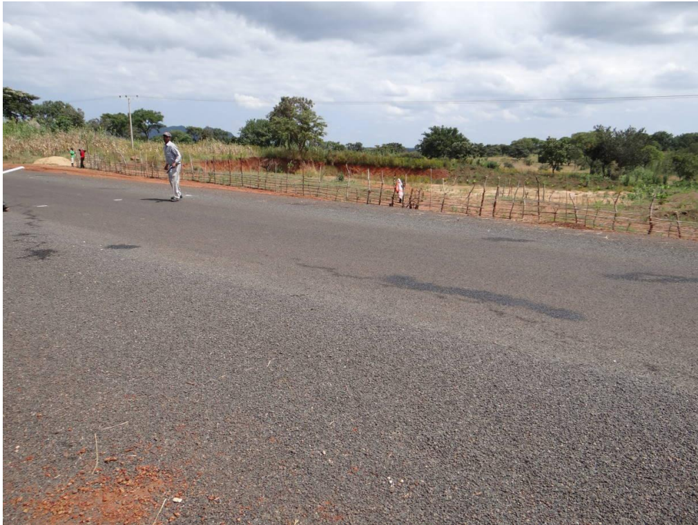
Figure 2-13 More spillage of petroleum products
