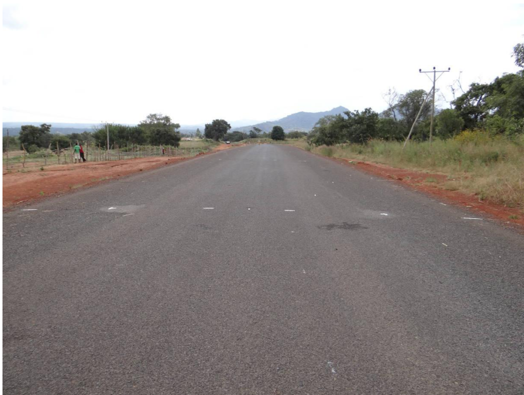
Figure 2-14 A section of the road with sealed shoulders
