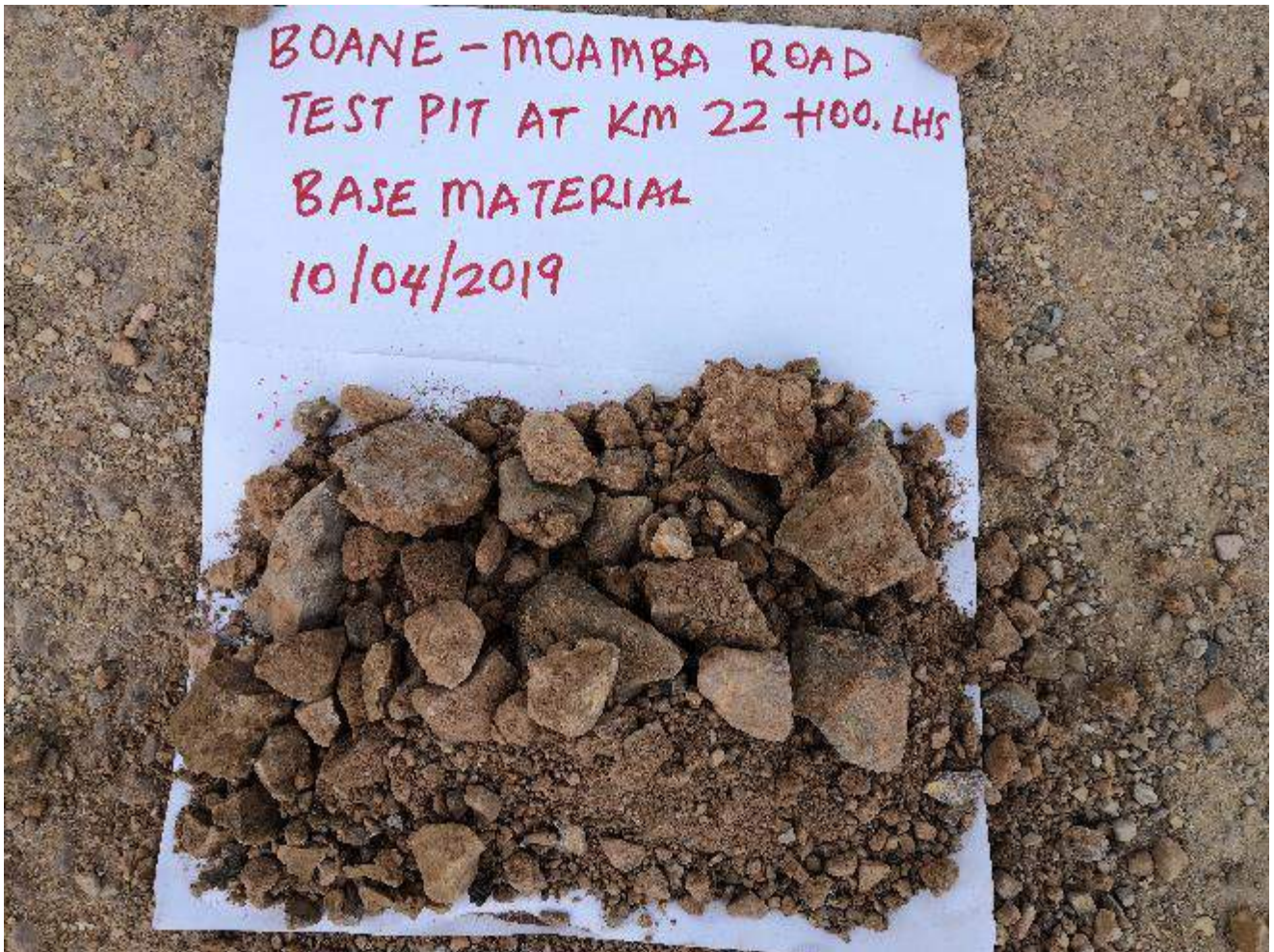
Figure 10 Base Course Boane – Moamba Section 1
