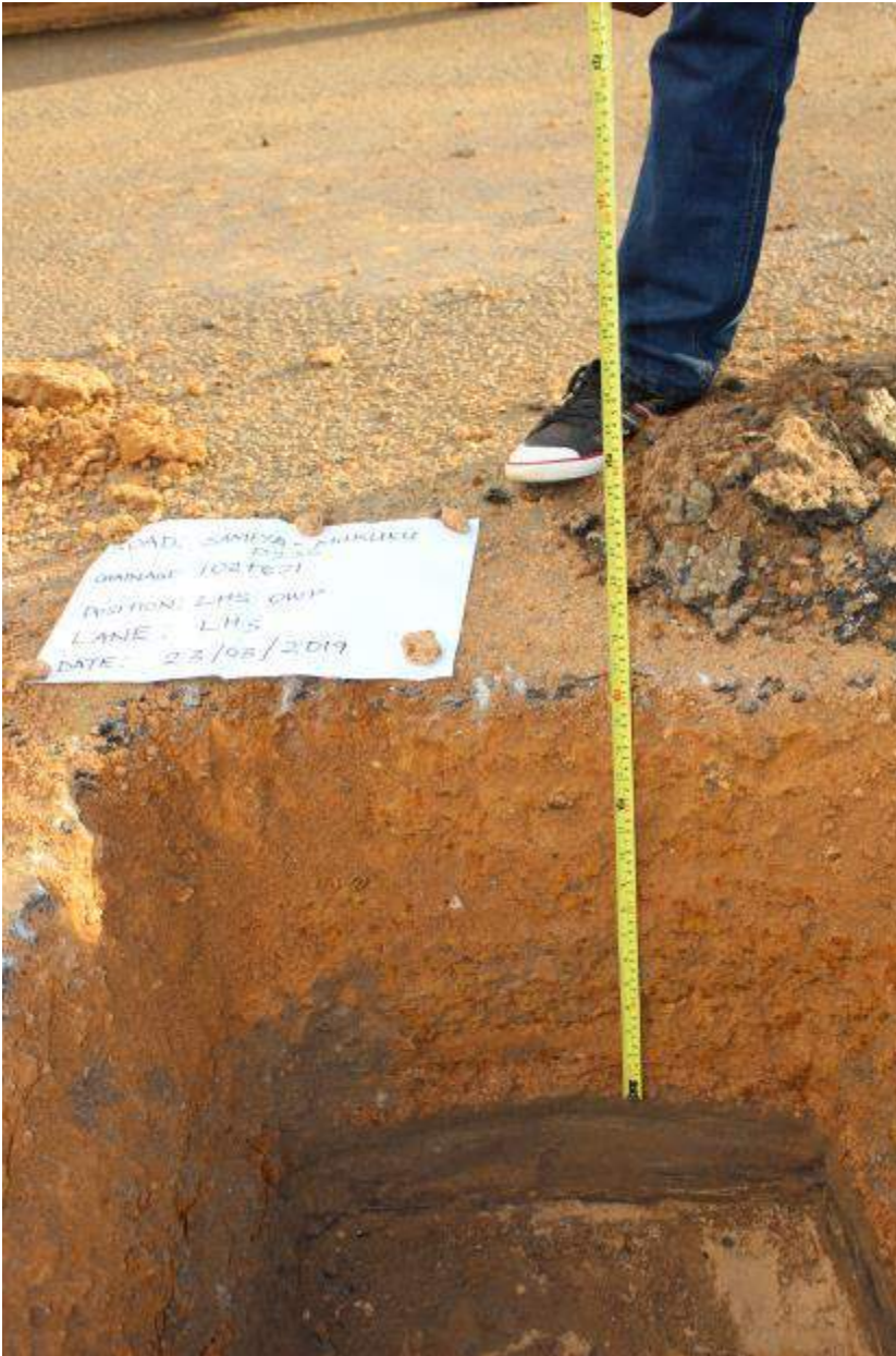
Figure 26 Test Pit on Section 2 Samfya – Mukuku Bridge road
