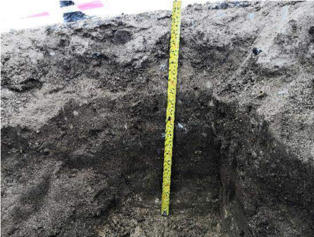
Figure 13 Test Pit on Section 2 Macia - Chokwe
