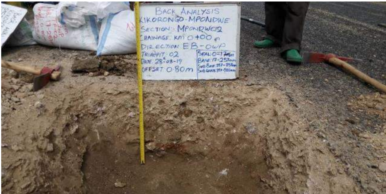
Figure 16 Test pit on Section 2 Kikorongo – Mpondwe
