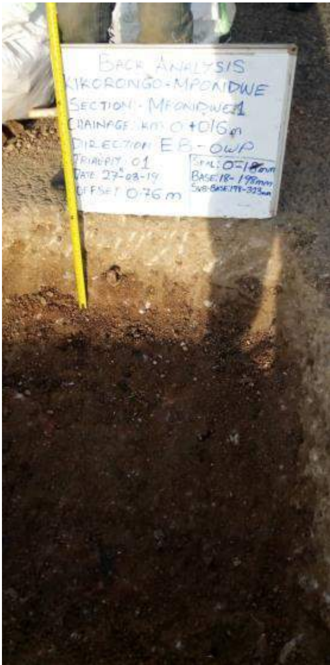
Figure 15 Test Pit on Section 1 Kikorongo – Mpondwe road
