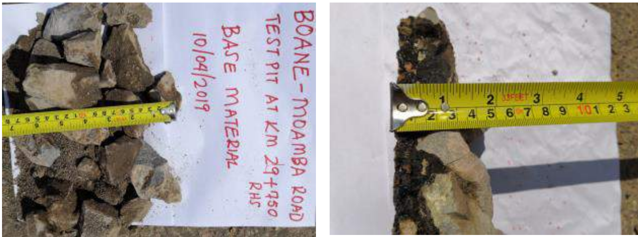
Figure 11 Coarse base materials and a well-bonded surfacing on Section 2 Boane - Moamba
