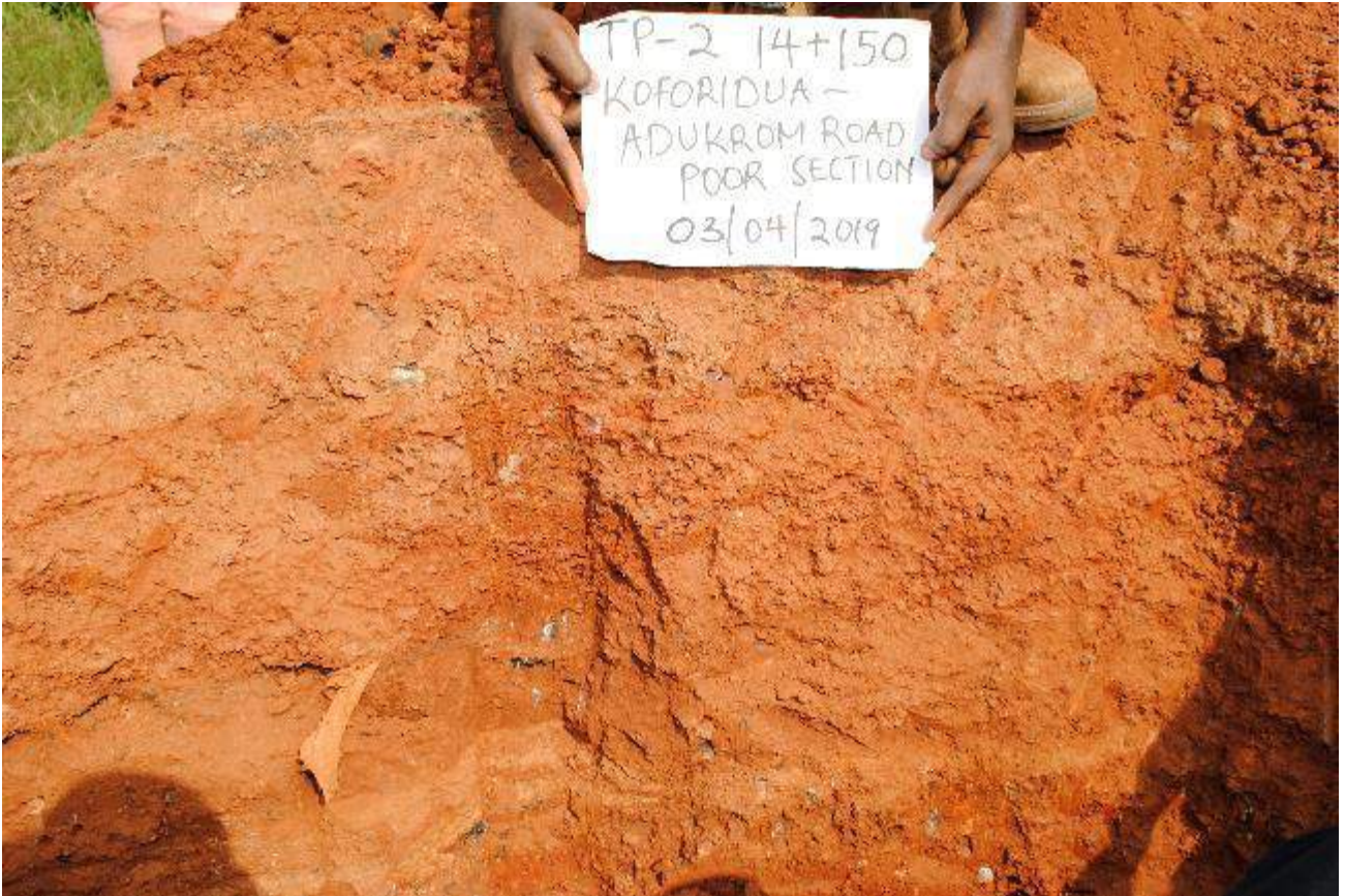
Figure 5 Test Pit on Section 1 Koforidua - Adukrom
