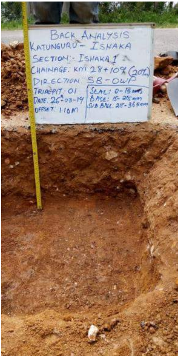
Figure 18 Test Pit on Section 1 Ishaka – Katunguru road
