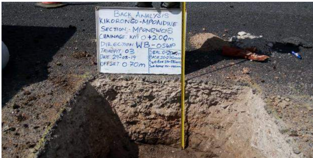
Figure 17 Test pit on Section 3 Kikorongo – Mpondwe
