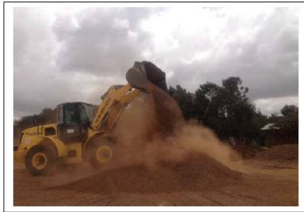
Figure 10 The front-end loader “airing” the aggregate in order to remove dust
