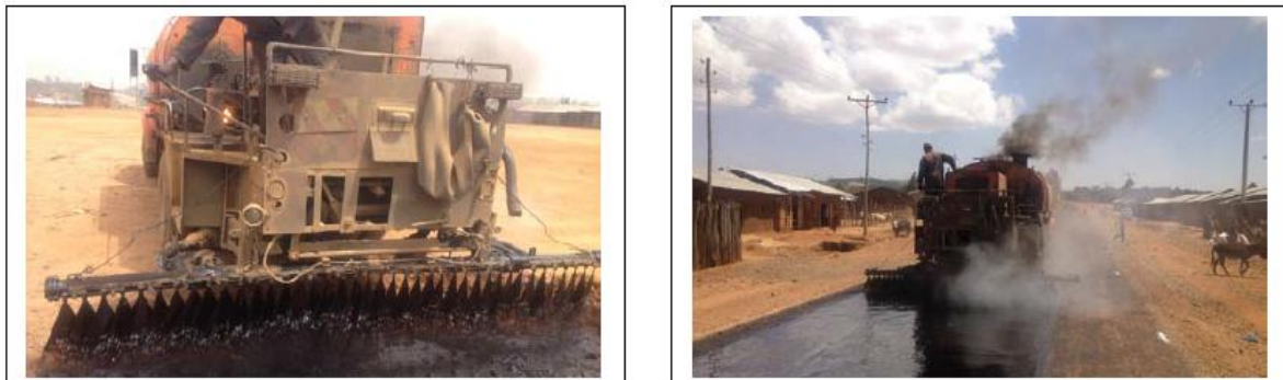
Figure 8 Checking the spray bar nozzels prior to spraying of binder
