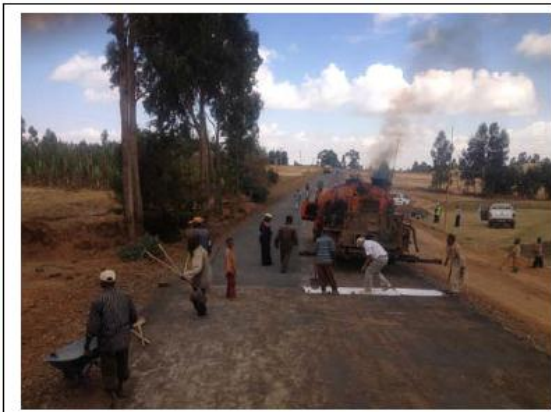
Figure 9 Paper laid to achieve straight transverse joints
