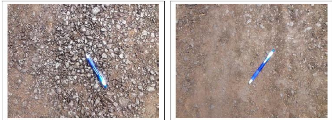
Figure 2 Coarse base and dense base layers after priming
