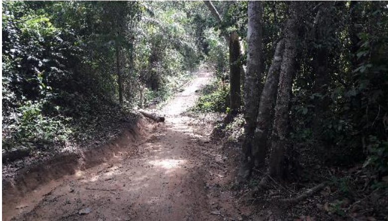
Picture 8 - A footpath to track upgrade in the Gogein area
