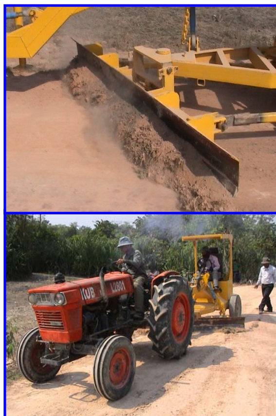
Figure 4 - ENGINEERED NATURAL SURFACES: Maintainable using simple locally made equipment
