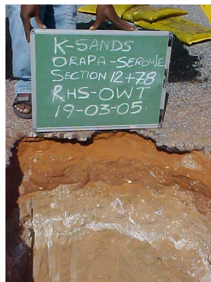
Plate 1—Kgalagadi sand roadbase & subbase on the Serowe-Orapa road
