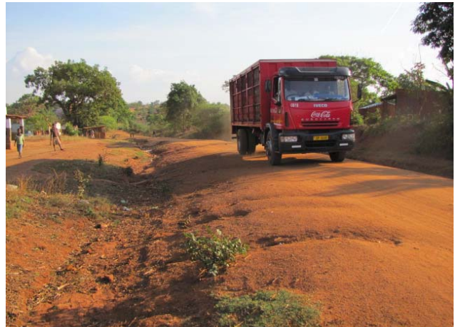
Section of gravel road on moderate gradient showing some rutting, deformation and drain erosion
