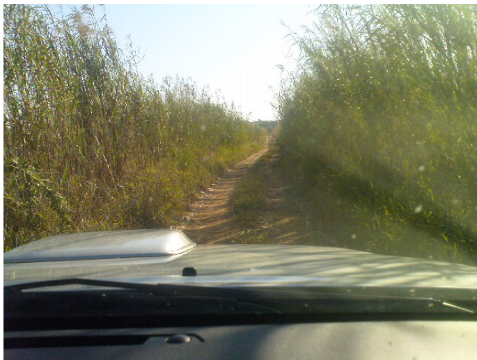
Route No R453: Combomune – Macandze – Gaza Province Condition: Poor
