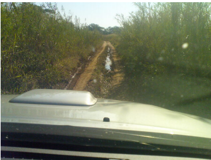
Route No R406: N200- Catuane - Maputo Province Condition: Poor
