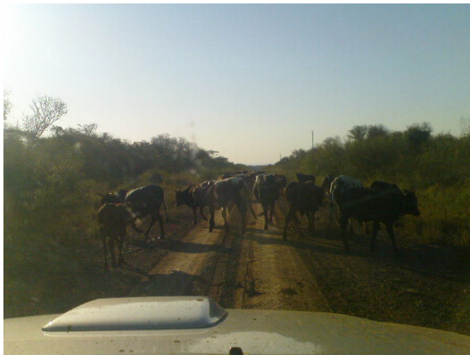
Route No R856: Chokwe – Fr Maputo – Gaza Province Condition: Poor
