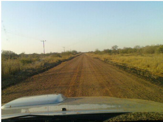
Route No N221: Macarante – Mabalane – Gaza Province Condition: Good
