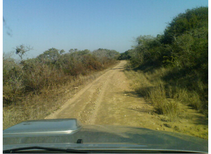
Route No: N200-Catuane – Maputo Province Condition: Poor
