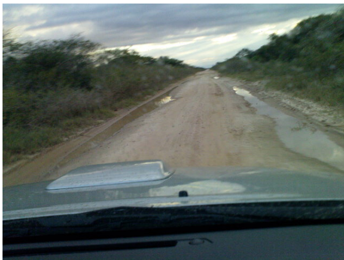
Route No: N221 Boane - Bela Vista – Maputo Province Condition: Good
