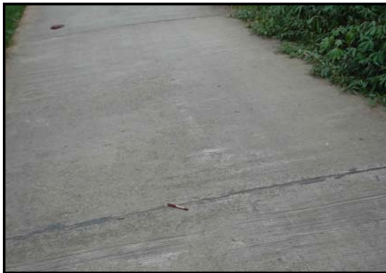
Figure 3.1 Full width concrete slab
