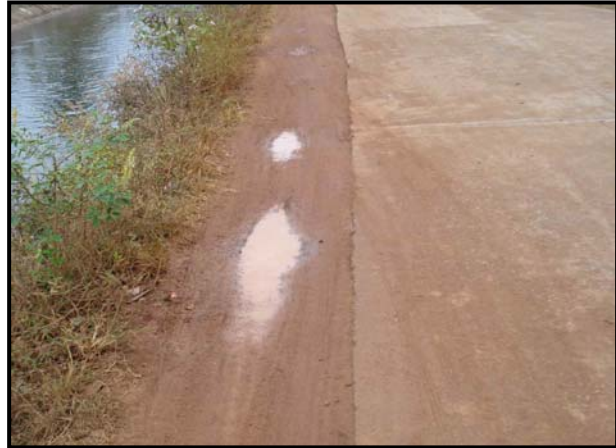
Figure 3.8 DL(3)-1. Saturated plastic shoulder gravel in contact with sub-base of same material. .
