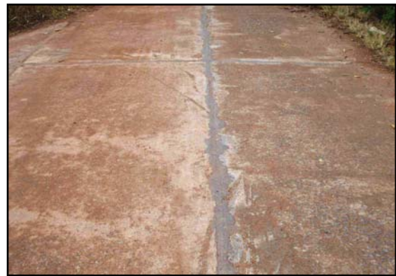
Figure 3.2 Half width concrete slabs
