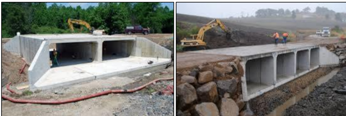
Figure 2-8: Structure monolithique - ponceau en caisson
