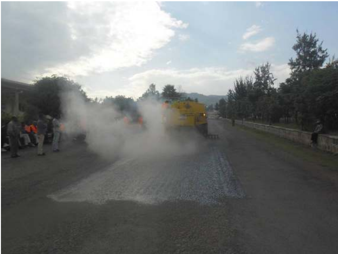
Figure 3-5 Longitudinal Spray Test
