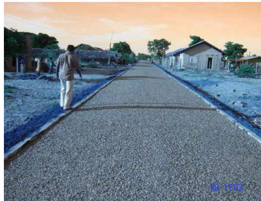
Photo 4: Completed road section
