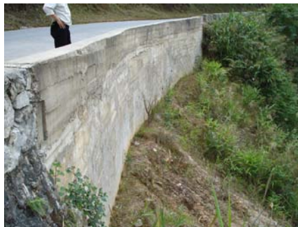
Reinforced concrete wall
