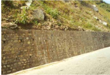
Mortared masonry wall
