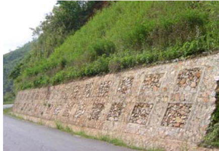
Composite masonry wall
