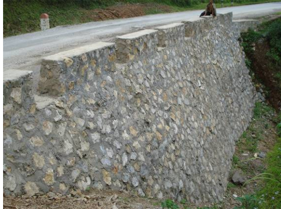
Mortared masonry retaining wall
