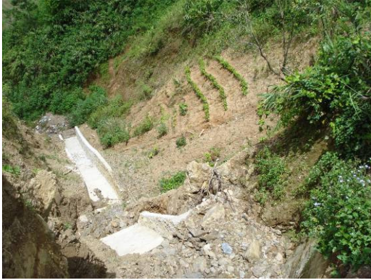
Mortared masonry channel
