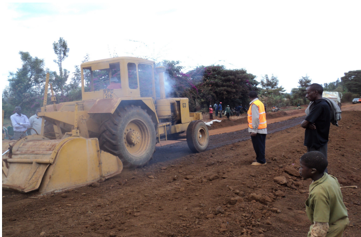
Plate 1: Mixing of Consolid system by Rotovator
