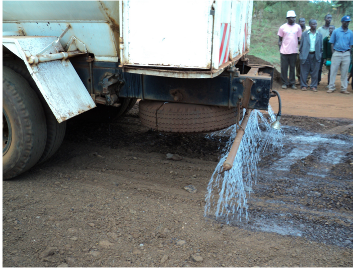
Plate 2: Application of Consolid C444 on sub base
