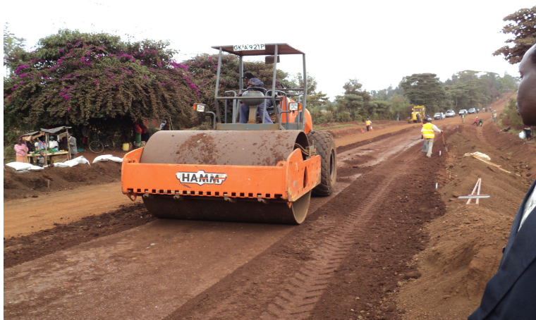
Plate 3: Compaction of Consolid system stabilized section
