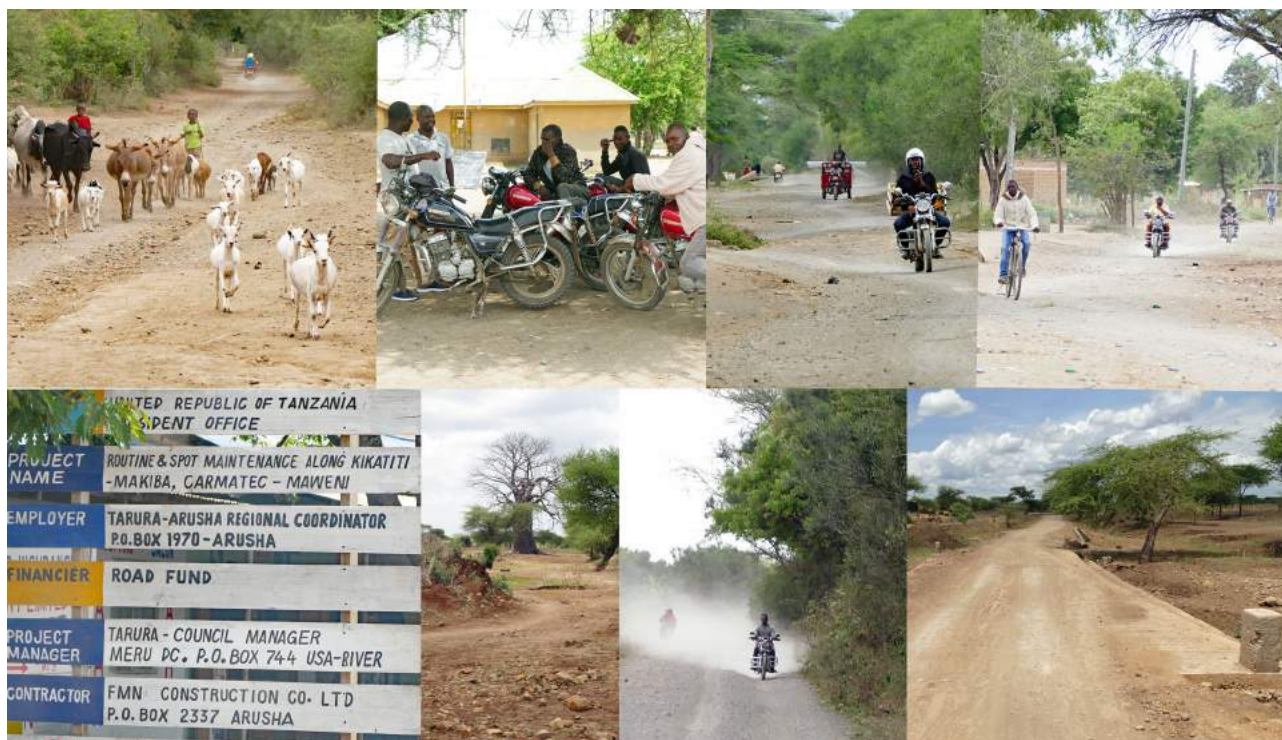
Figure 4 Photo montage illustrating some aspects of the Matiba Road
