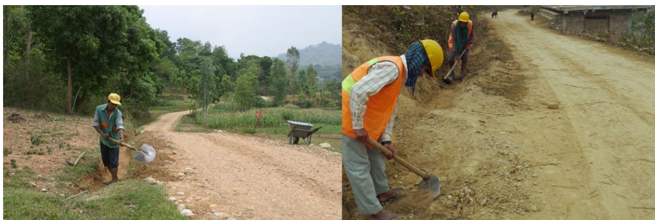
Figure 16 Lengthworkers maintaining earth roads in Nepal
