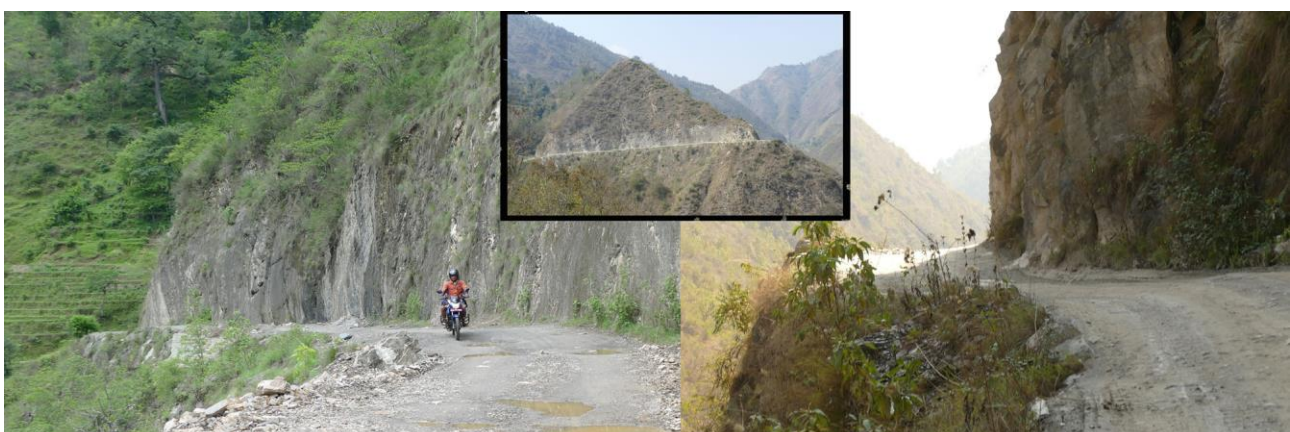
Figure 10 Earth sections on the Kavre road studied in Nepal that have allowed buses to operate for ten years
