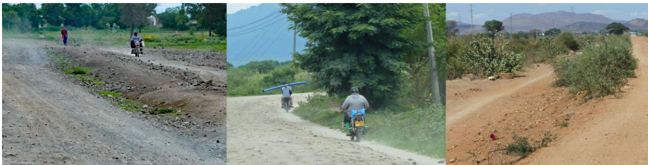
Figure 12 Examples of side trails that have developed on three of the surveyed roads in Tanzania
