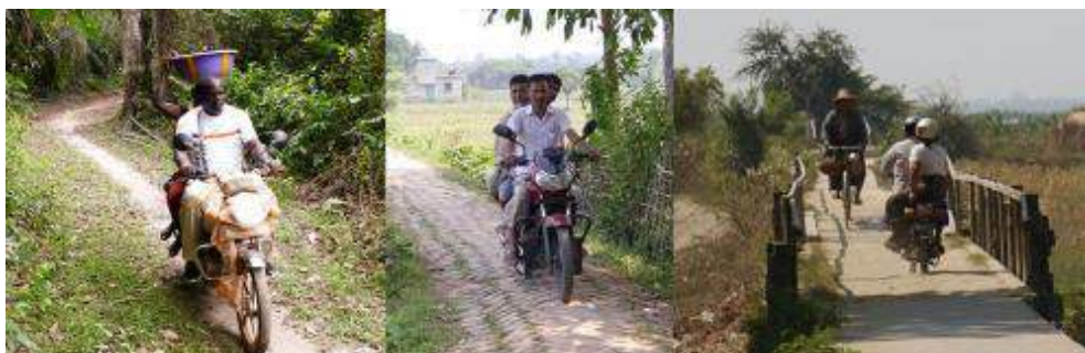
Figure 119 Examples of constructed motorcycle trails in Liberia (left), Bangladesh (centre) and Myanmar (right)
