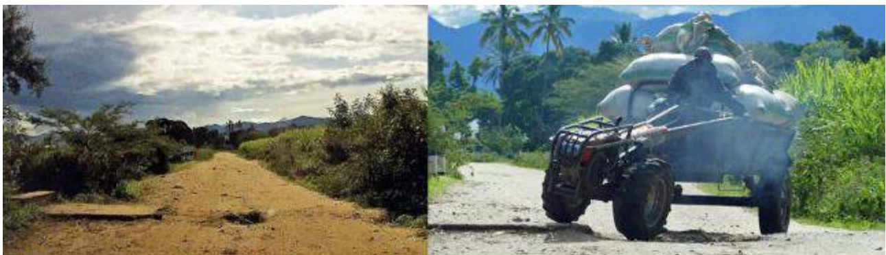
Figure 36 A broken culvert showing a two-wheel tractor negotiating the problem
