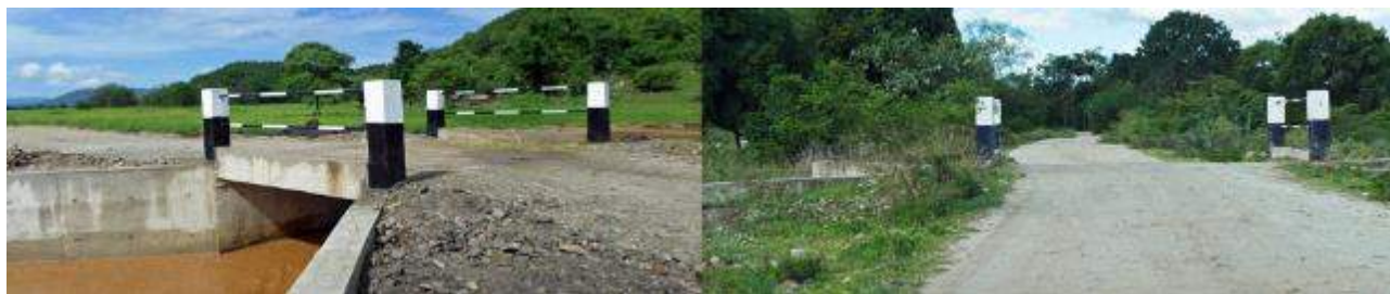
Figure 33 IRAT box culvert immediately after completion in 2016 (left) and in 2019 (right)
