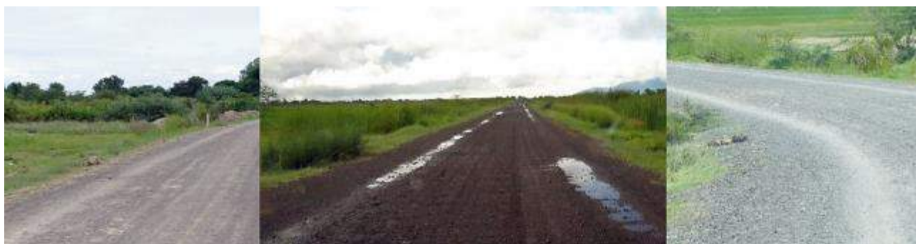
Figure 21 Gravel road surface showing puddles (centre) and smooth tracks worn by motorcycles (left and right)
