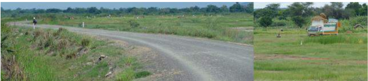
Figure 13 Chekimaji to Kawaya road showing raised embankment through rice-growing swampy area
