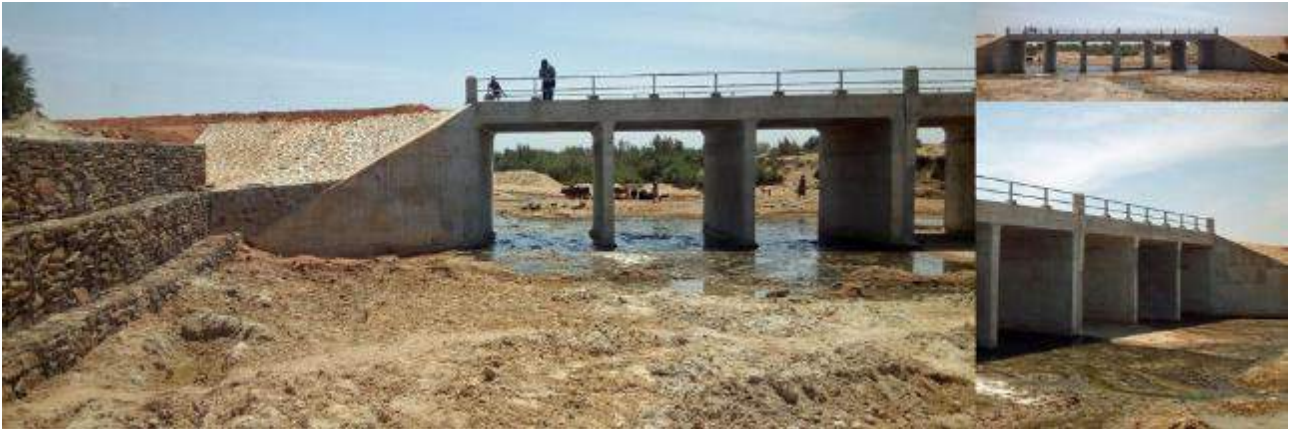
Figure 51 Chigongwe-Chipanga Road Bridge 1 (6-cell box culvert) after construction
