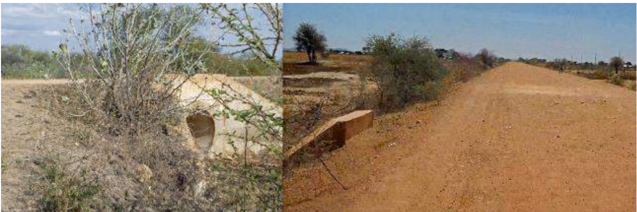
Figure 72 Mpunguzi-Mwitikira road showing ring culverts included in the IRAT investments
