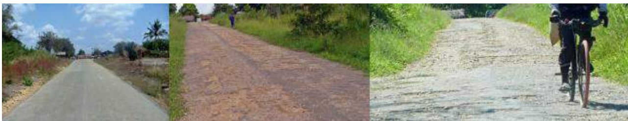
Figure 111 Slurry seal section in 2011, 2015 and 2019
