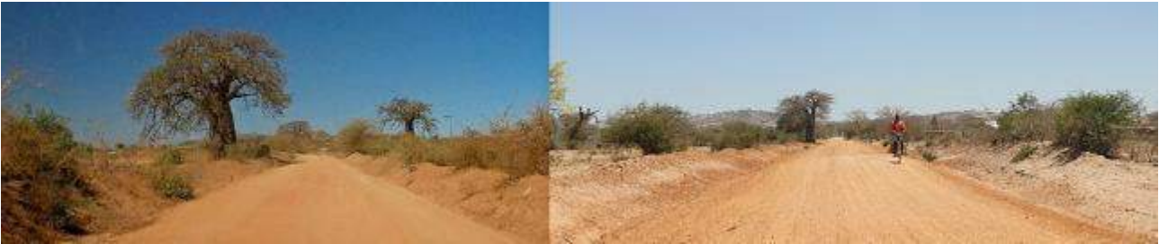
Figure 57 Chigongwe-Chipanga road showing a well-maintained shape
