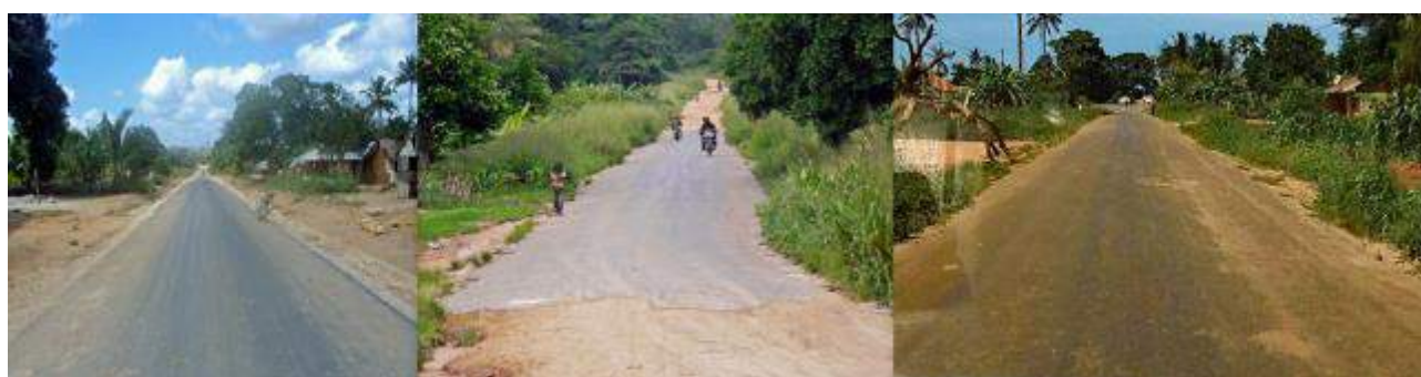
Figure 100 Otta seal section near Bago in 2011, 2015 and 2019 (L-R)
