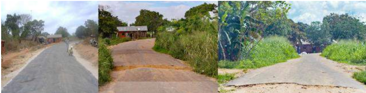
Figure 109 The double sand seal section in 2011 (left), 2015 (centre) and 2019 (right)
