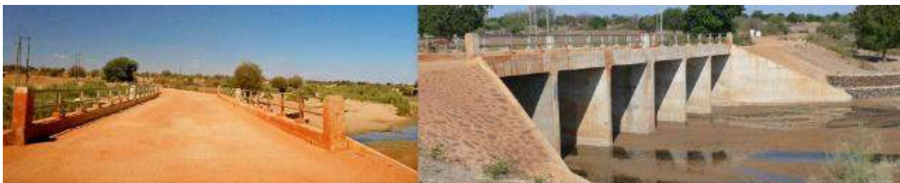
Figure 60 Chigongwe-Chipanga road Bridge 1 (6-cell box culvert)
