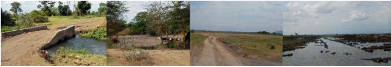
Figure 11 Chekimaji to Kawaya road before construction, including in the rainy season (right)
