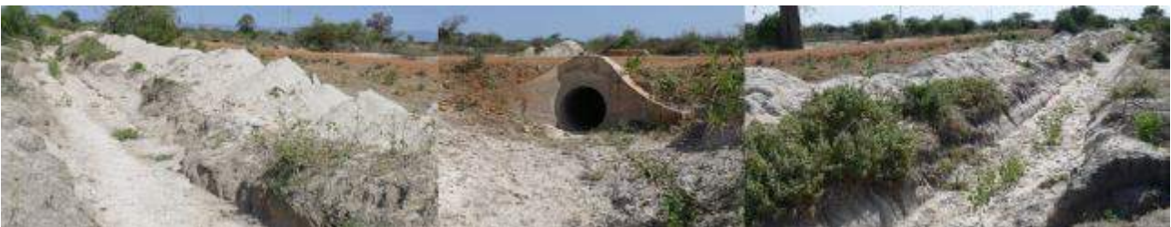
Figure 58 Chigongwe-Chipanga road showing side drains to catch run-off from the land
