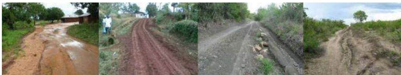
Figure 97 Examples of road condition in 2009 before AFCAP1 intervention
