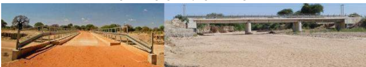
Figure 61 Chigongwe-Chipanga road Bridge 2
