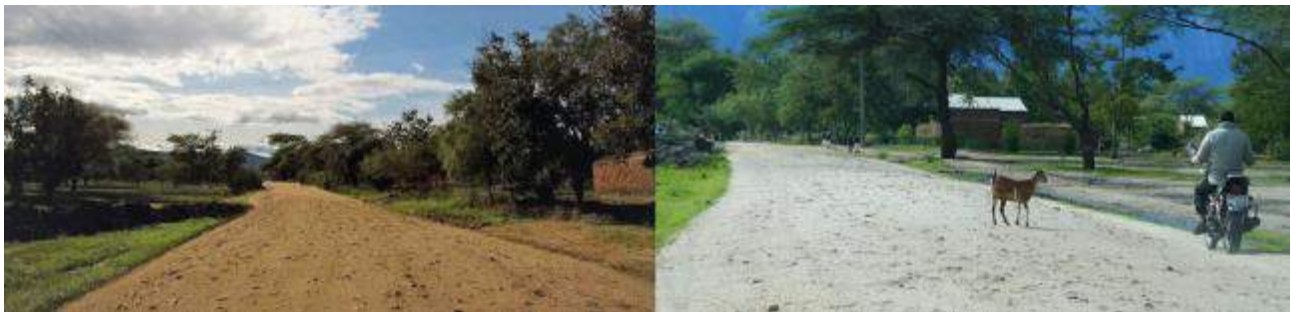
Figure 35 The first section of the road, showing oversize stone causing a rough surface that motorcycles avoid
