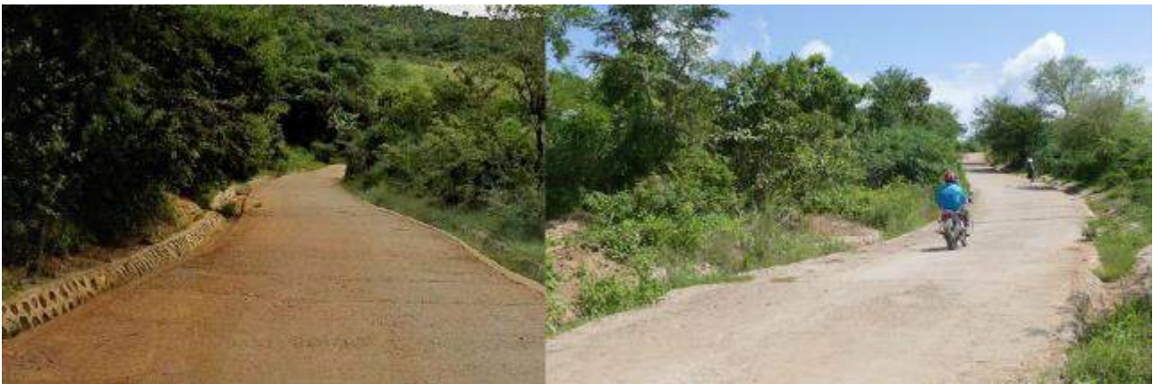
Figure 89 Concrete section on the Mikese-Ngeregere road in 2019
