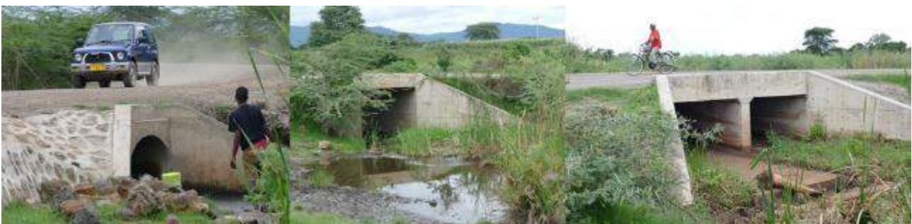
Figure 14 Three of the culverts included in the IRAT rehabilitation
