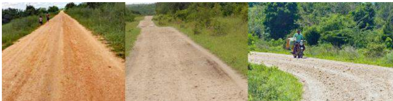
Figure 101 Gravel sections in 2011 (left), in 2015 (centre) and 2019 (right)
