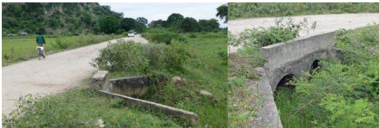
Figure 38 IRAT-funded culverts, showing vegetation growing in the silt
