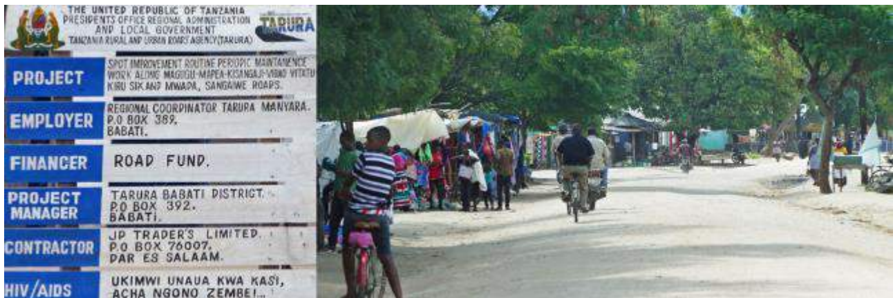
Figure 34 TARURA maintenance sign (left) and first section of the road close to Magugu (right)
