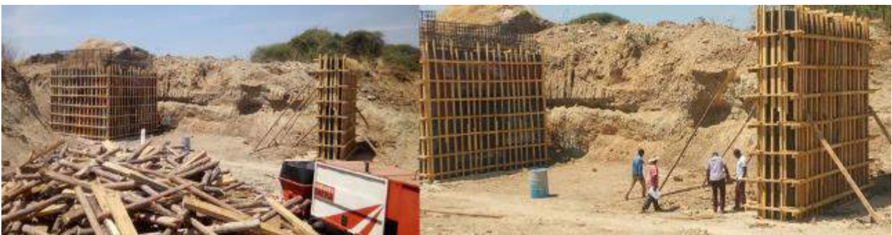
Figure 52 Chigongwe-Chipanga Road Bridge 2 during construction
