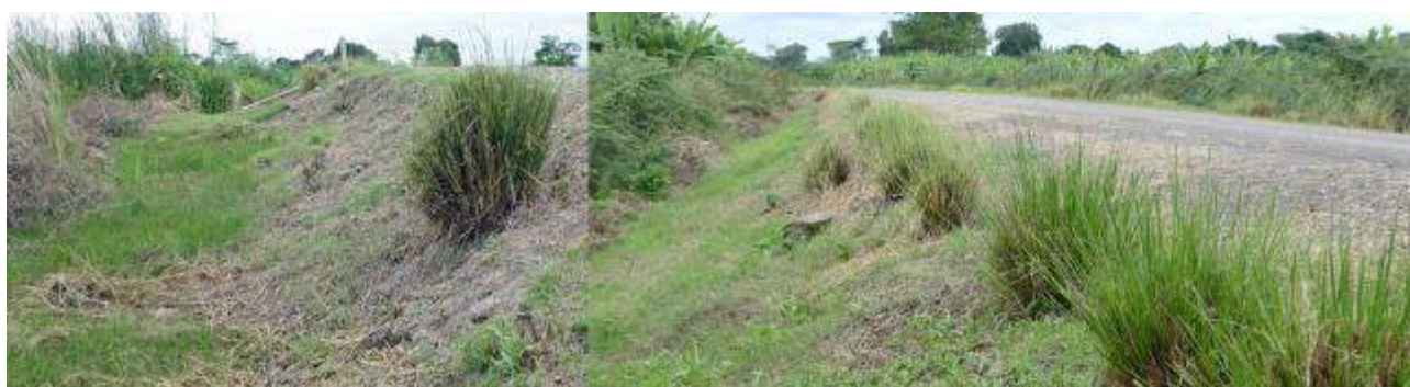
Figure 22 Road embankment showing vetiver grass planted for erosion control
