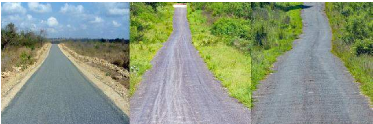
Figure 108 The double surface dressing section in 2011 (left), 2015 (centre) and 2019 (right)
