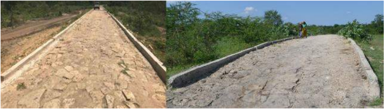
Figure 104 Re-habilitated packed stone section in 2016 (left) and 2019 (right)
