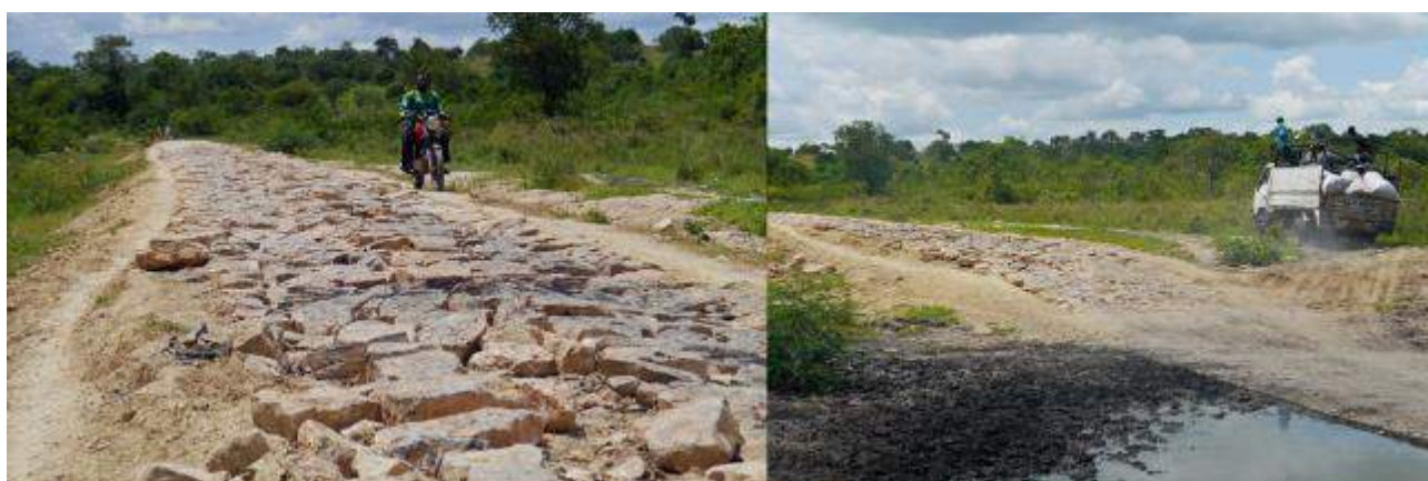
Figure 103 Transport responses to failed section showing motorcycle shoulder trails and truck on side trail
