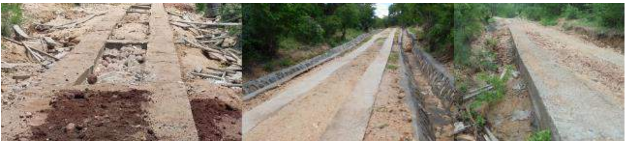
Figure 84 Parallel concrete strips constructed under IRAT rehabilitation interventions in 2015
