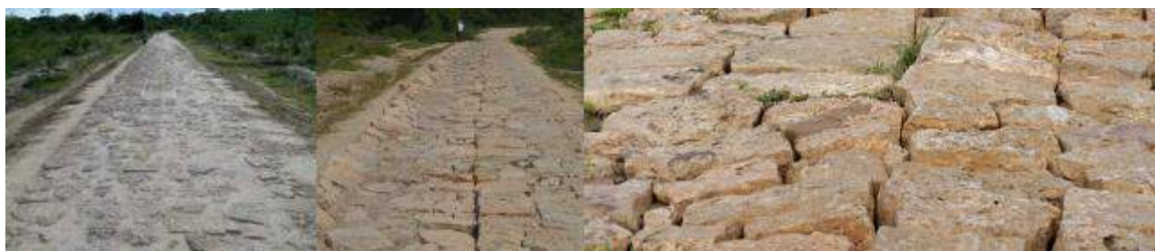
Figure 102 Hand-packed stone section in 2011 (far left), in 2012 (centre) and 2015 (right)
