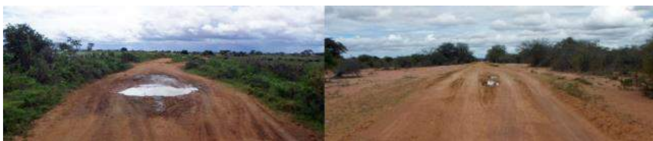
Figure 68 Mpunguzi-Mwitikira road in 2015 prior to IRAT rehabilitation
