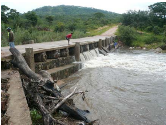
Improved structure on Rio Nhimbe with water flowing at both levels
