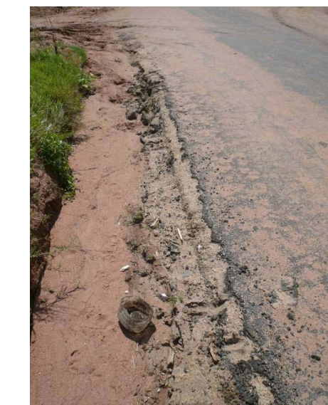
Section 3: Erosion and reduced lateral support
