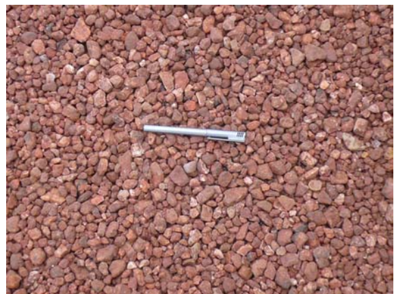
Newly constructed Otta seal – detail
