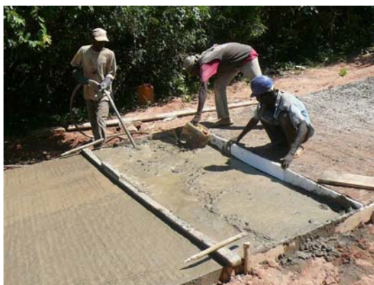
Concreting a slab
