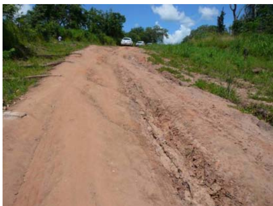
Eroded section of road prior to the main ramp
