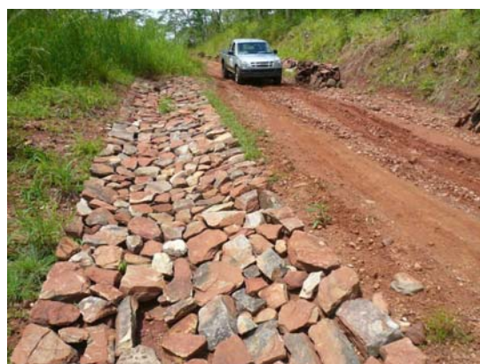
Preparation of mortared stone pitched side drain
