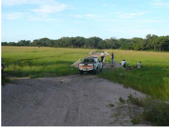
Swamp crossing with two culverts
