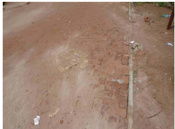
Section 1: Surface detail
