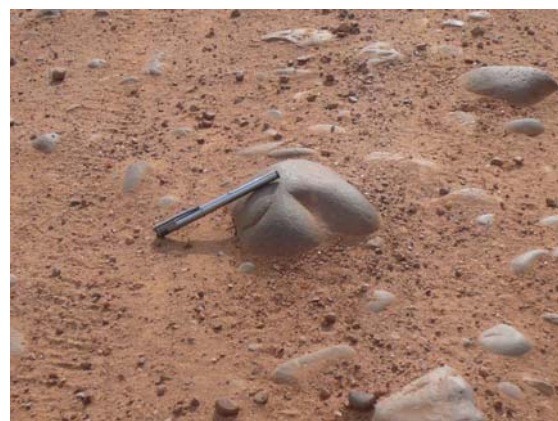
Rough surface of the original road – detail
