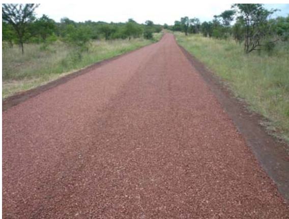
Newly constructed Otta seal
