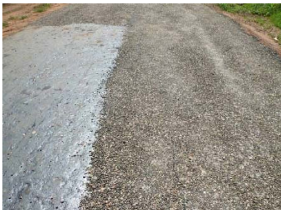
Section of prime (L) and Cape seal (R)
