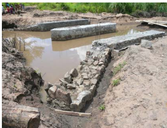
Culvert approximately 19 km from Gracio under construction
