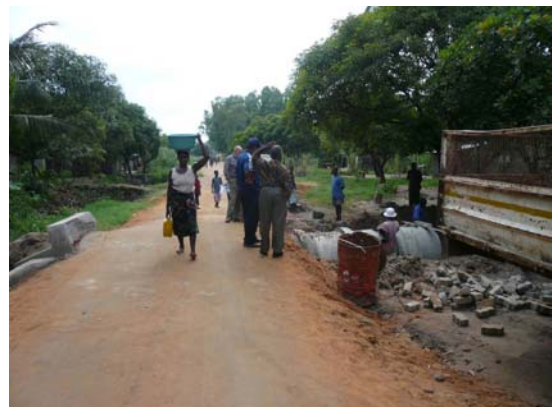
Raised culvert construction in the urban area
