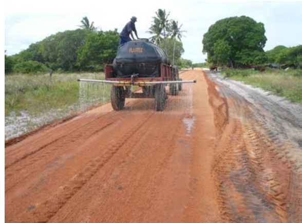
Completed red sand gravel beyond the RRIP funded improvements
