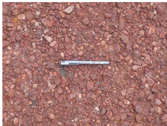
Otta seal after initial rolling
