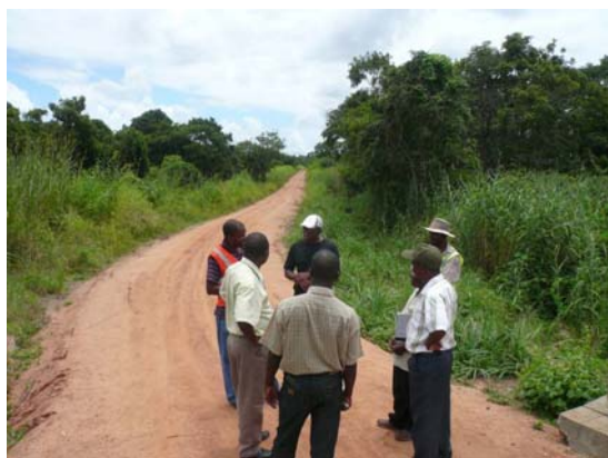
Section, beyond Mecuburi bridge, which is said to overtop
