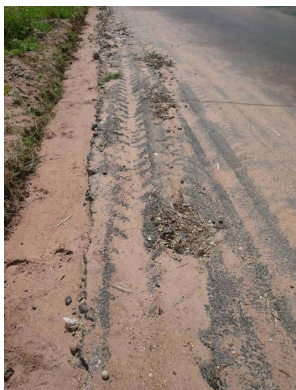
Section 3: Left hand side edge damage
