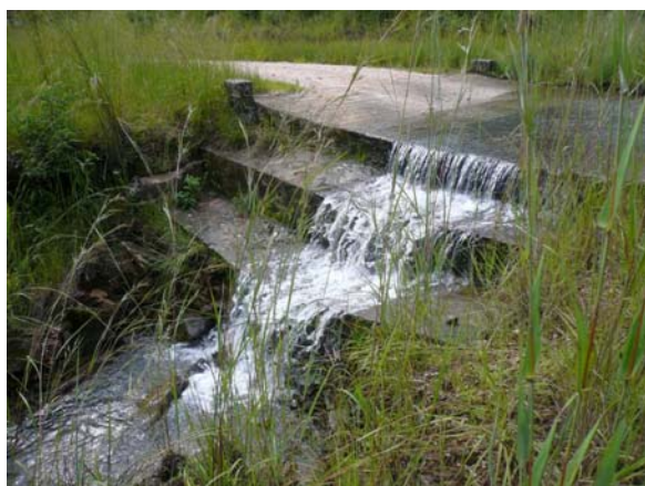
Well designed drift outlet
