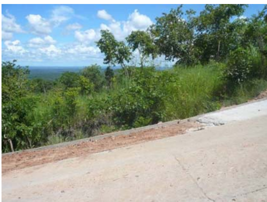
View across a steep section of the ramp
