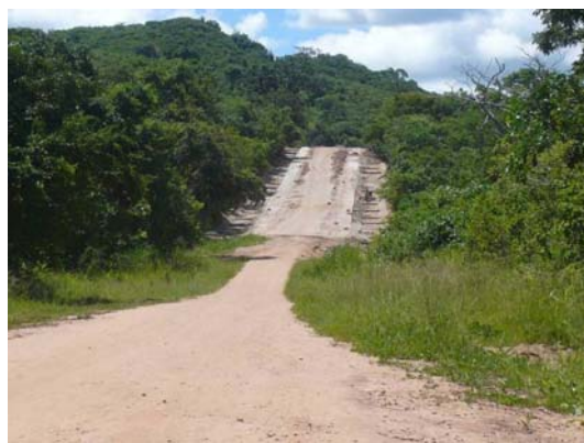
Toe of the concrete surface on the main ramp
