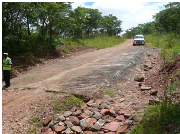
Short trial section of surfacing
