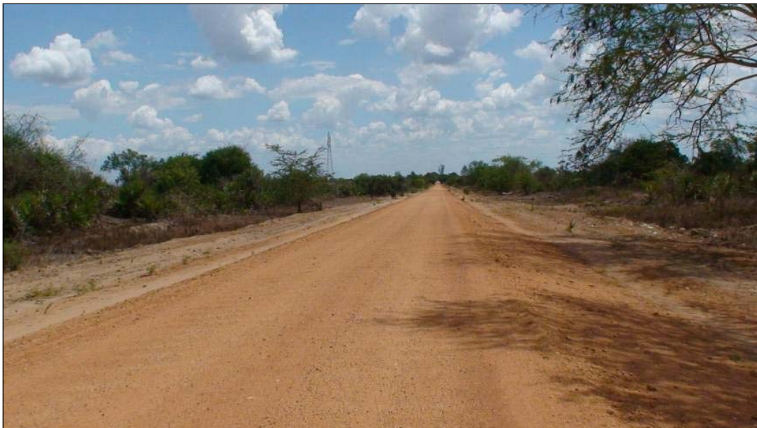
Section of the completed Zero Mopeia road
