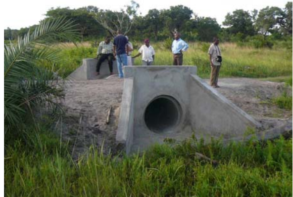
Short access ramps up to soffit level
