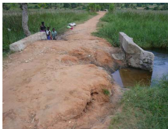
One of several original culverts to be cleaned and repaired
