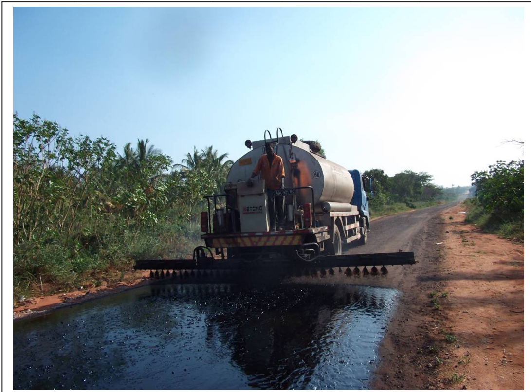
Figure 4-8 Binder application and illustration of blocked nozzle
