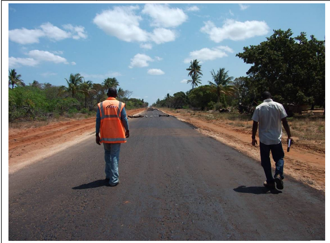
Figure 4-5 Primed section ready for Otta seal surfacing
