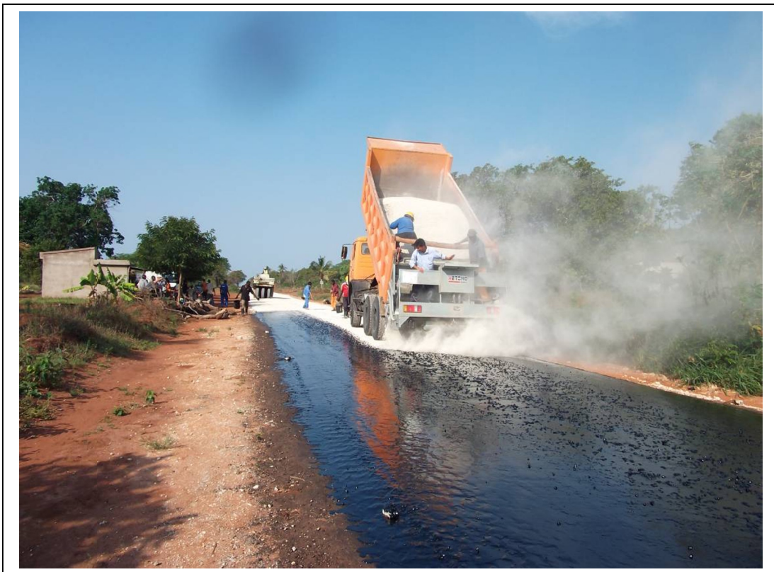
Figure 4-6 Dusty calcrete aggregate
