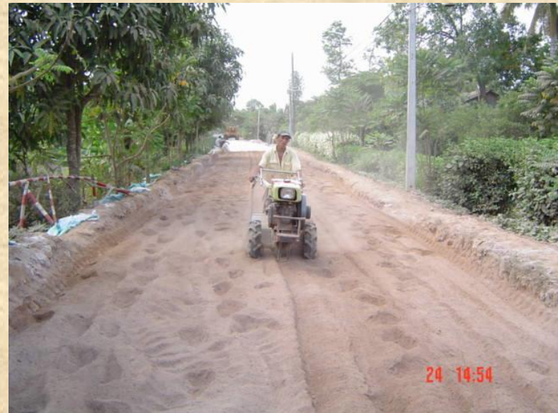
e.g. Construction of lime stabilised roadbase
