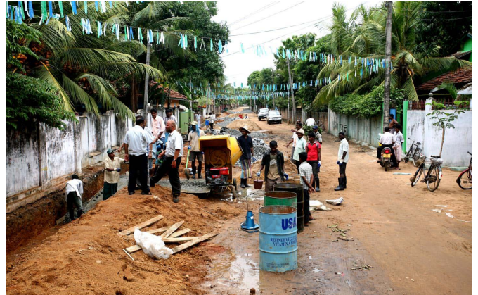
Road works in progress in rural Sri Lanka
