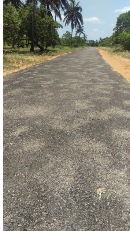
Toward end of construction
