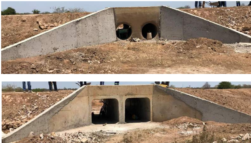
Figure 1.19 Extension of wing walls of the existing culverts at km 43 (western side)
