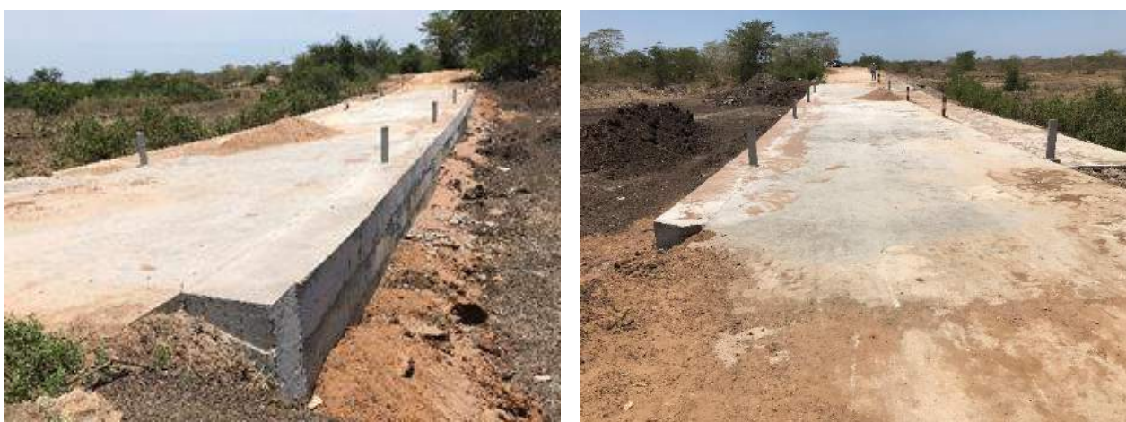
Figure 1.9 General view of the completed wall
