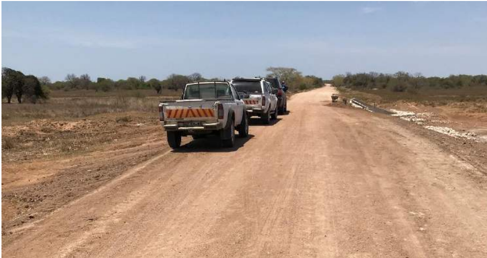
Figure 1.18 General view of approach road (existing culverts at km 43)
