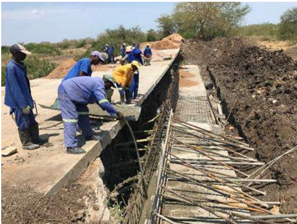
Figure 1.7 Concrete pouring and vibrating
