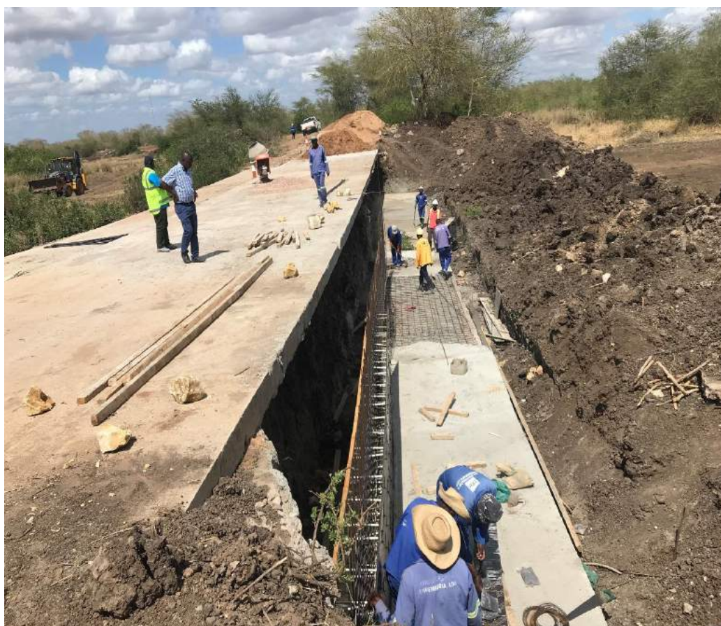
Figure 1.3 Formwork preparation and reinforcing steel fixing km 17.6)
