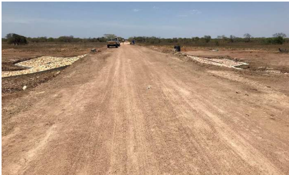
Figure 1.16 General view of approach road (new culvert at km 43)
