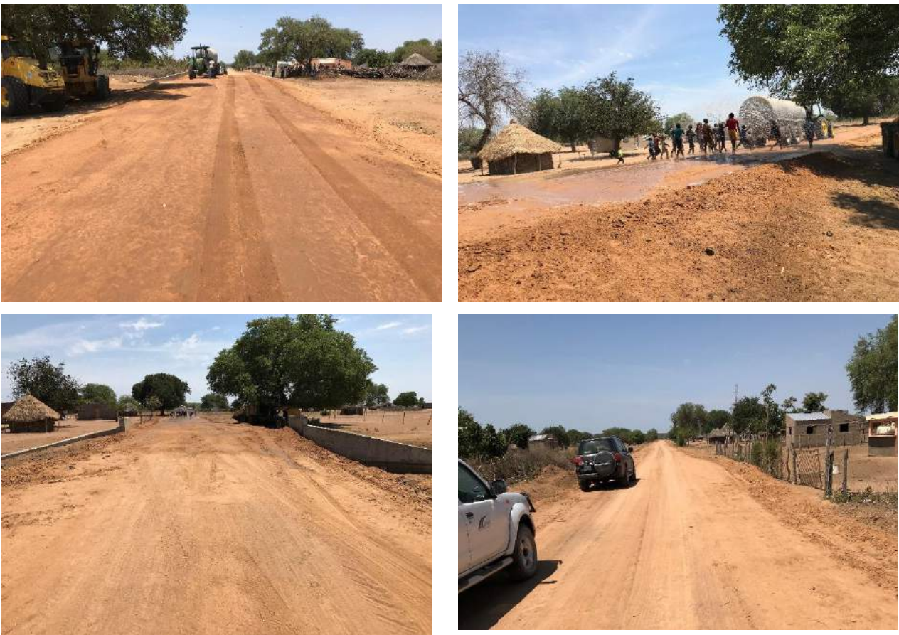
Figure 1.22 Progress on the construction of the improved road at km 51
