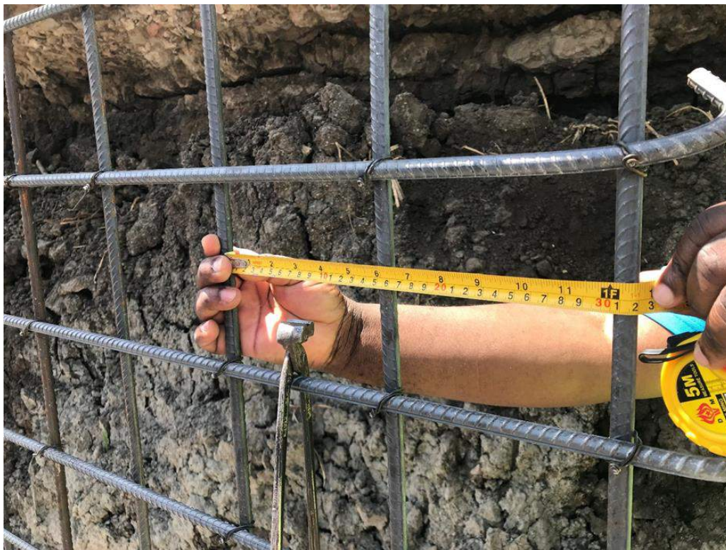
Figure 1.5 Verification of reinforcing steel spacing
