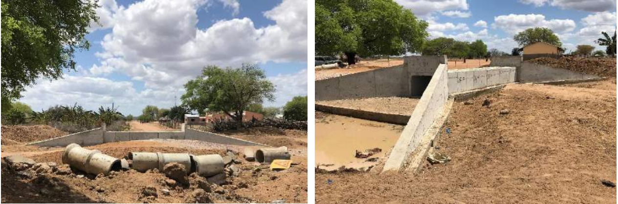
Figure 1.21 Construction of the a new culvert at km 51
