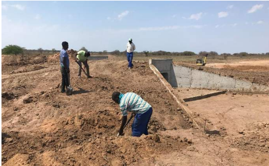
Figure 1.15 Construction of erosion protection (new culvert at km 43)
