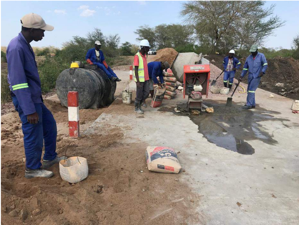
Figure 1.6 Concrete mixing
