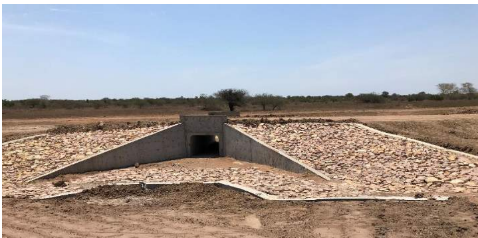
Figure 1.17 Erosion protection (stone pitching and beam) for new culvert at km 43)
