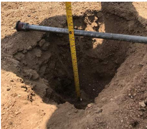
a) Closer to the concrete ford (300 mm)
