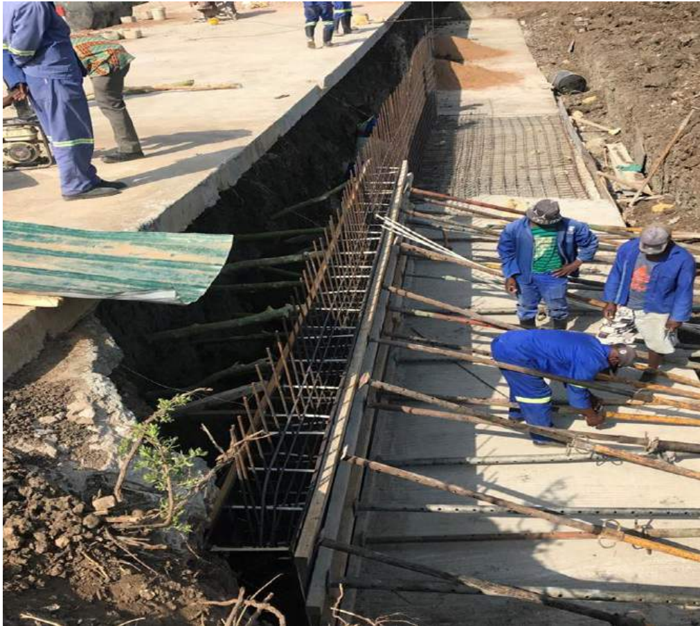
Figure 1.4 Installation of formwork support
